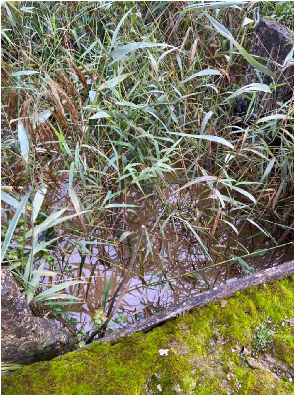
Figure 2. Culvert inlet looking westwards towards open channel
