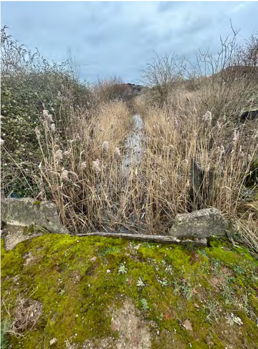
Figure 1. Culvert inlet looking westwards towards open channel
