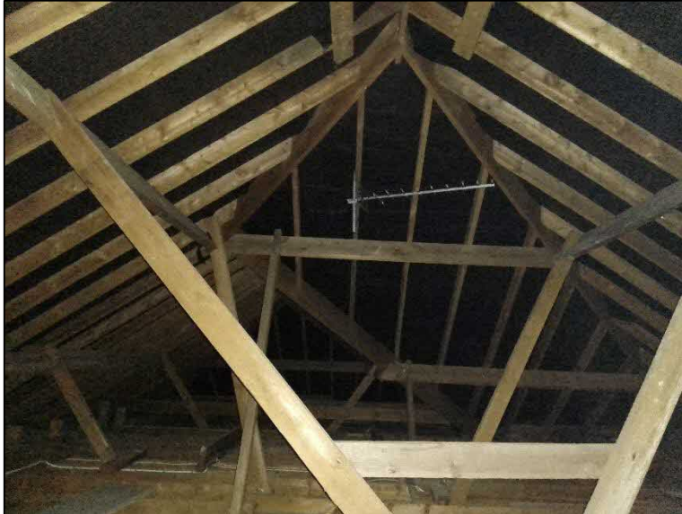
Photograph 2– Example view of the void interior.
