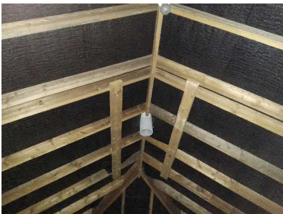
Photograph 5 – Example view of the pipe in the ridge.
