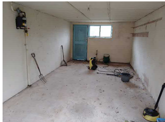
Photograph 4 – View of the garage interior.
