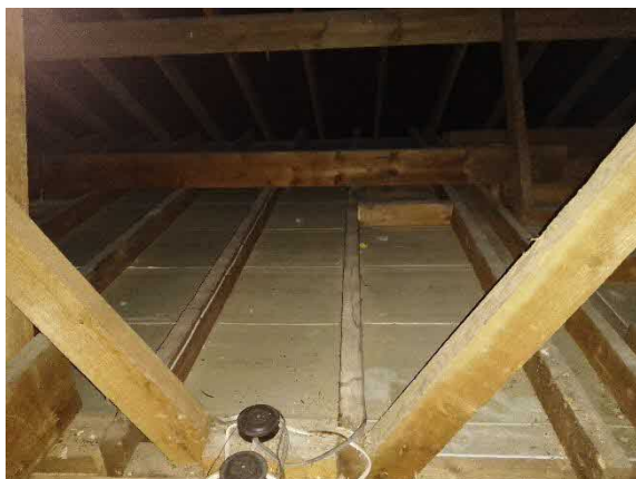
Photograph 6 – Additional view of void floor.
