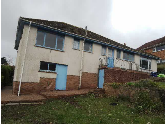
Photograph 1 – View of the north aspect.
