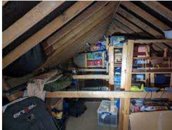
Photo 3. Showing the roof void over the house
