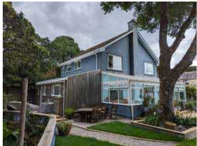
Photo 2. Showing the house from north west
