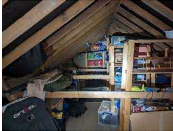
Photo 3. Showing the roof void over the house
