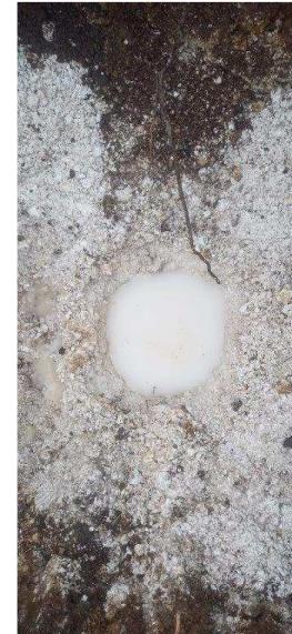
Percolation test (BS6297) in progress
