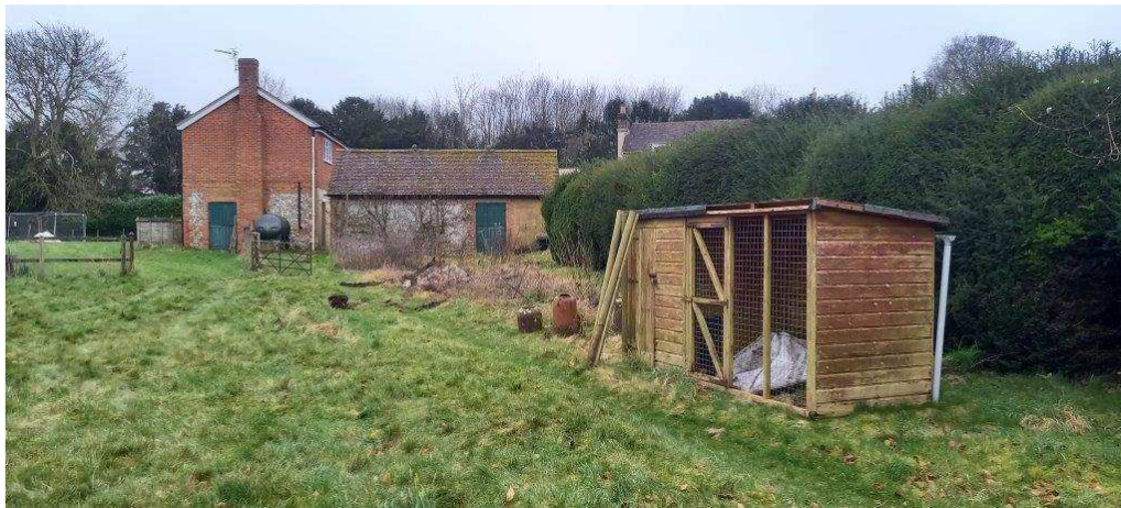
View of the site from the west
