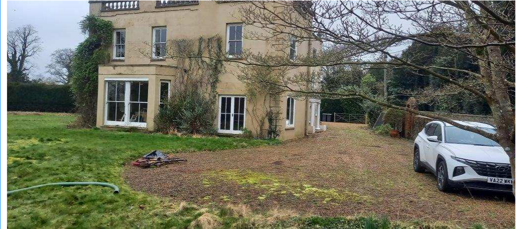
View of the existing 3-storey building from south-east
