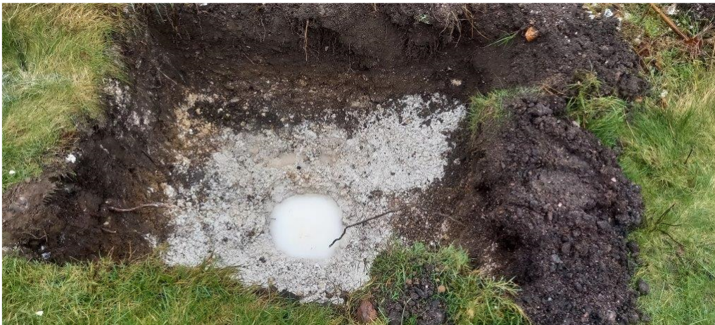
Percolation test (BS6297) in progress
