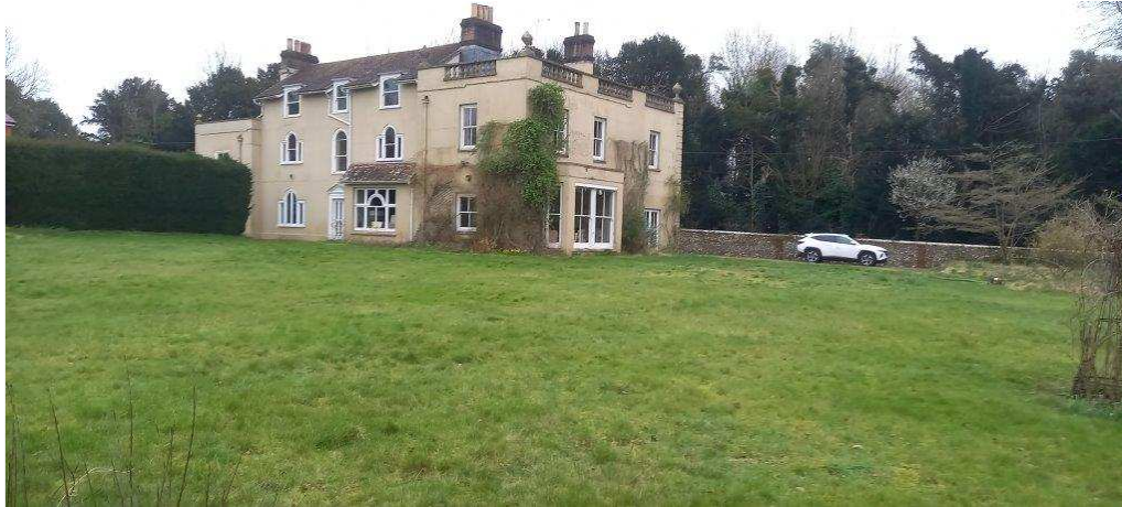
View of the existing 3-storey building from south
