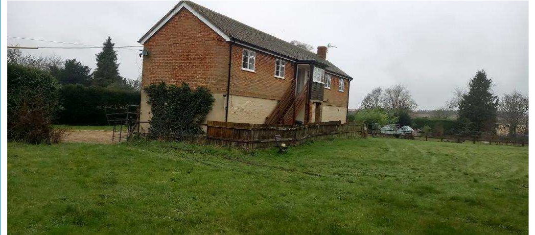
View of the 2-storey building
