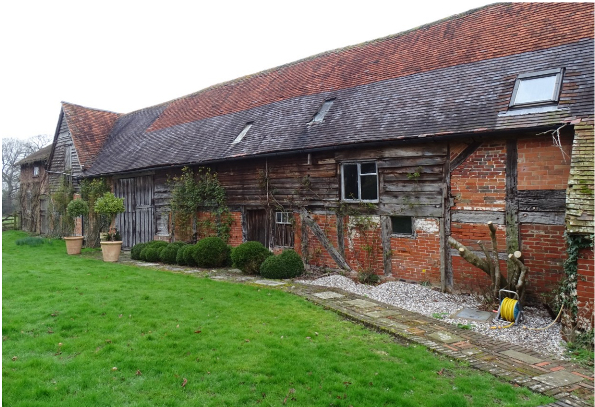
Image 16 – B1 – South facing elevation of the structure
