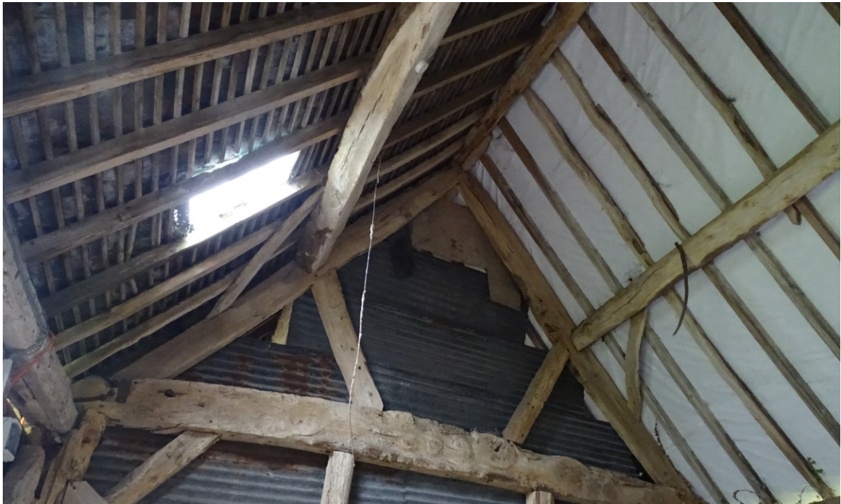
Image 20 – B1 – Internal view from within the structure
