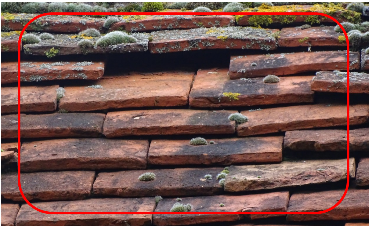
Image 17 – B1 – Examples of gaps with the South facing roof coverings of the structure which looks to offer shelter/access opportunities for both bats and nesting birds
