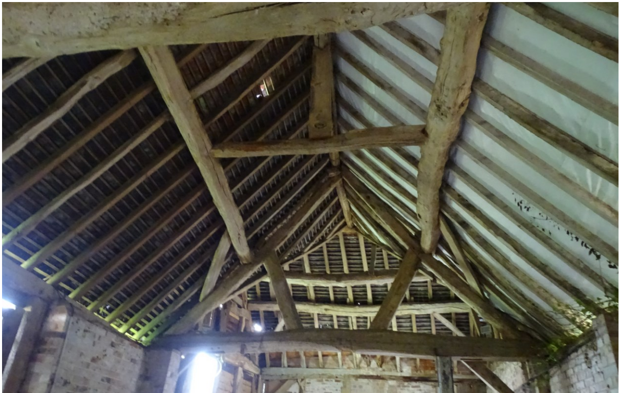
Image 19 – B1 – Internal view from within the structure
