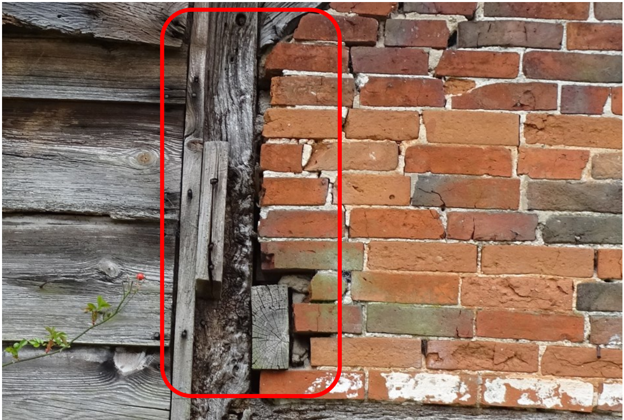
Image 18 – B1 – Examples of gaps within the South external brickworks which looks to provide further opportunities for bats
