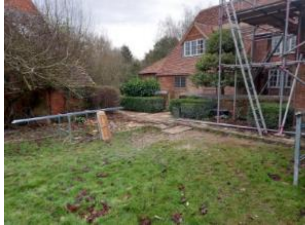
Plate 3.9: View of northern elevation of house and pathway
