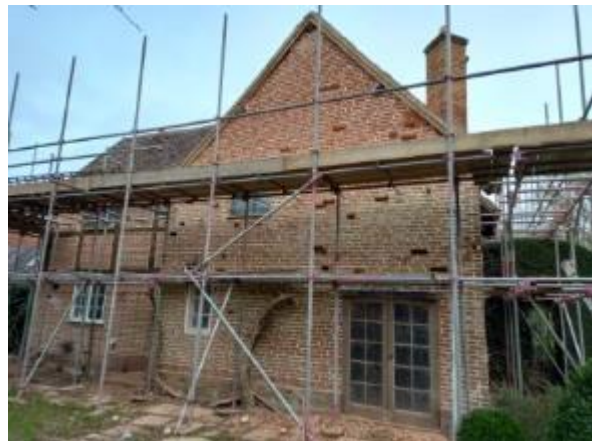
Plate 3.2: Western end of existing house showing repair works and patio/path
