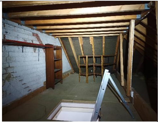
Photograph 4: Storage loft above the single storey extension
