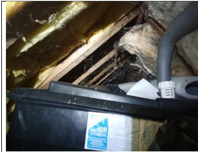
Photograph 3: Roof void in the apex of the main house
