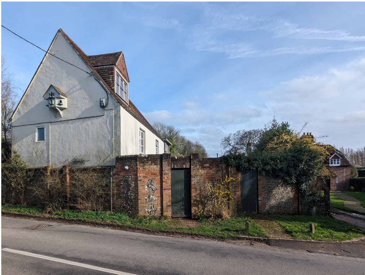
Photograph of the existing brick and flint wall from the Droxford Road
