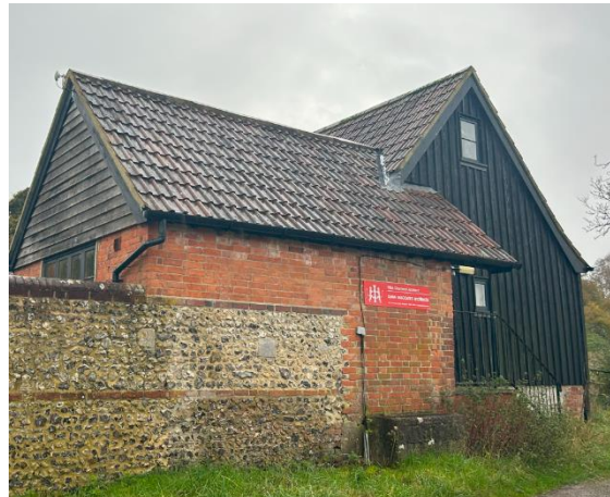
Figure 3 – Examples of vertical board and batten cladding used within the local area
