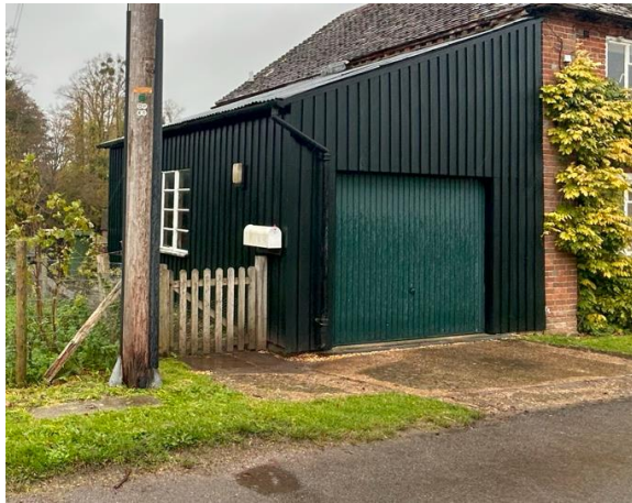
Figure 3 – Examples of vertical board and batten cladding used within the local area
