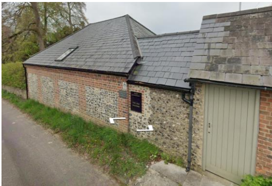
Figure 2a – The Old Rectory, Rectory Lane
