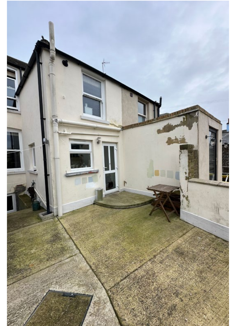
Rear of the property showing existing extension of neighbouring building.
