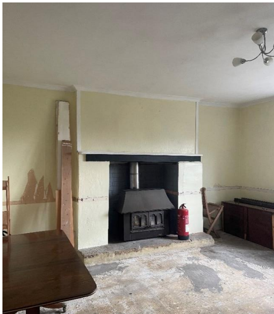
FIG 35: GF NORTH N-S WING RECEPTION ROOM FIREPLACE
