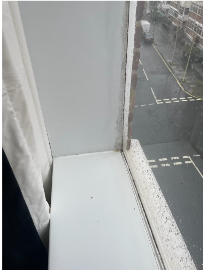
Picture 3: Existing Window
