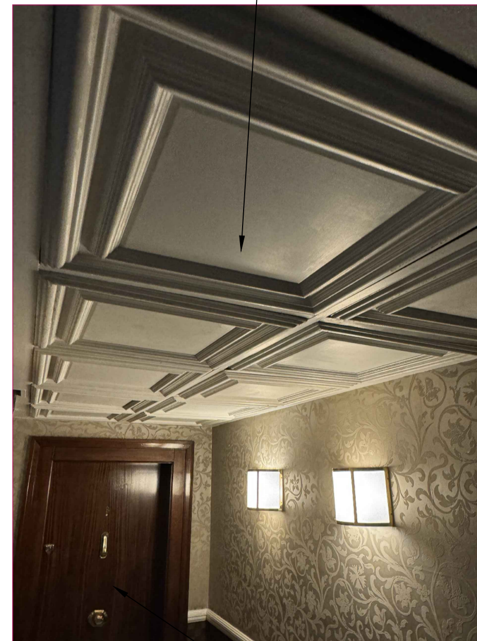
FLAT ENTRANCE DOOR TO BE REPLACED
