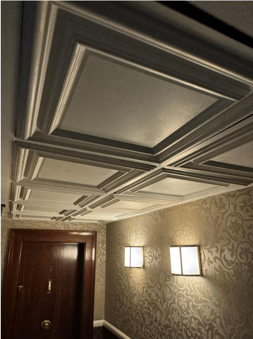
Photograph 4 – Suspended ceiling at lower ground level
