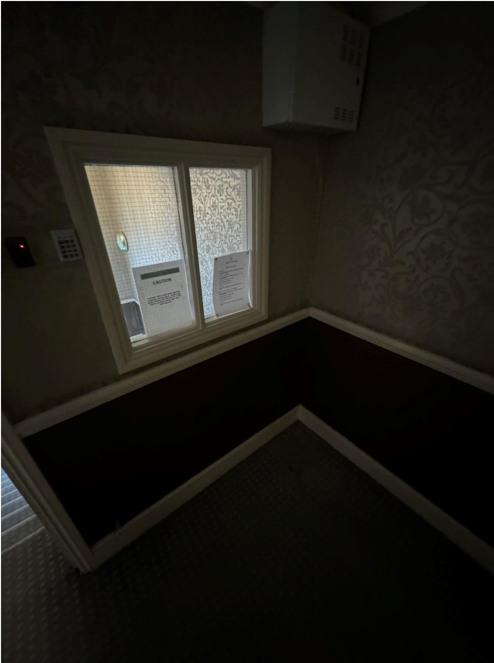
Photograph 8 – Timber stud wall at fourth floor
