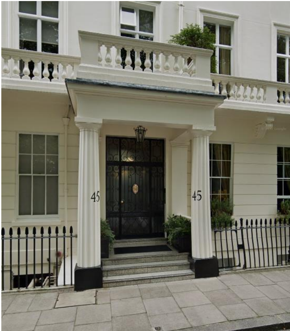
Photograph 10 – Existing Terrazzo / Tiled finish to front entrance steps.
