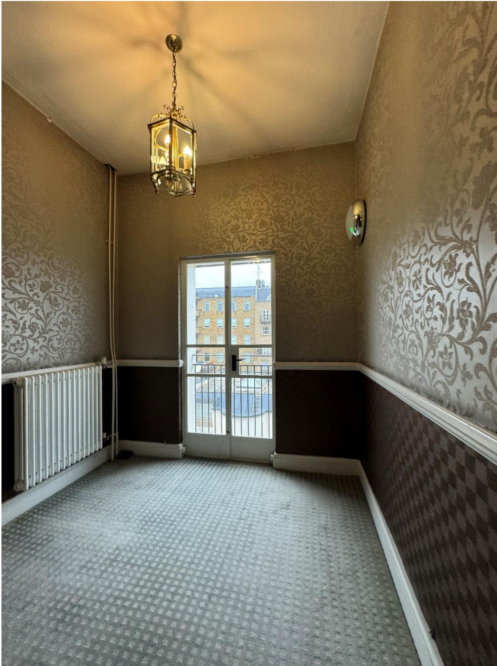
Photograph 7 – Existing Crittall door to rear elevation
