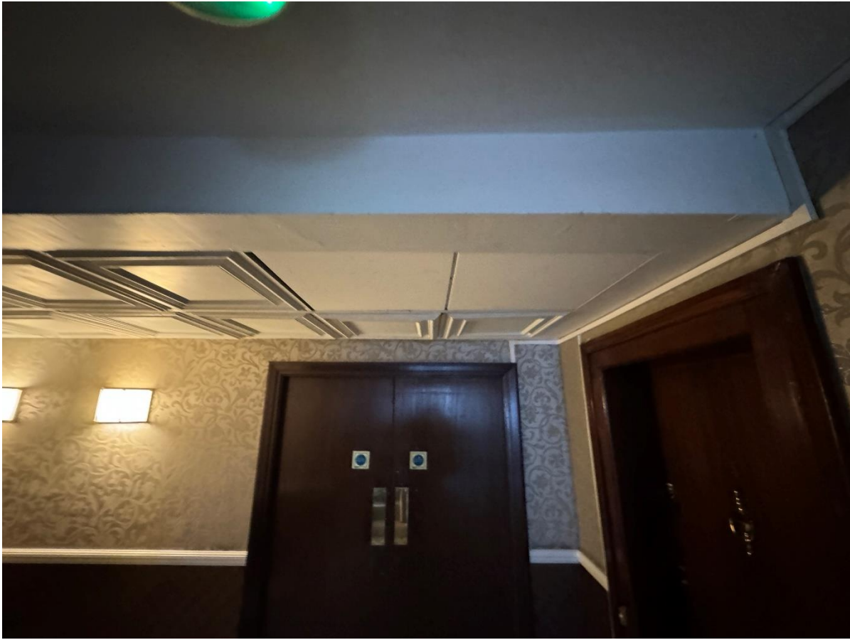
Photograph 5 – Suspended ceiling at lower ground level
