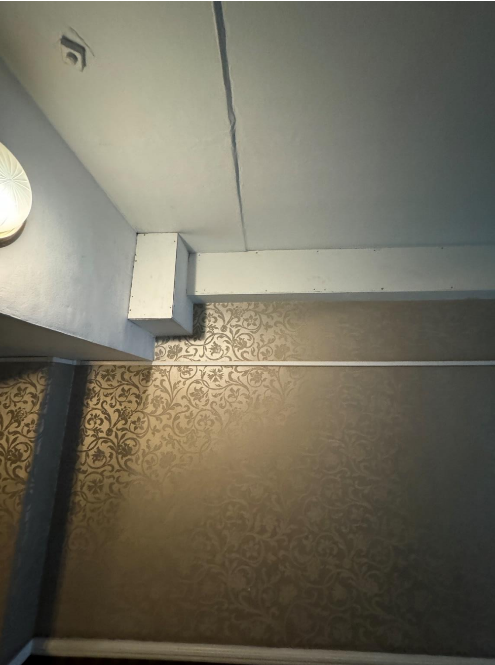
Photograph 3 – Existing boxing at lower ground level.
