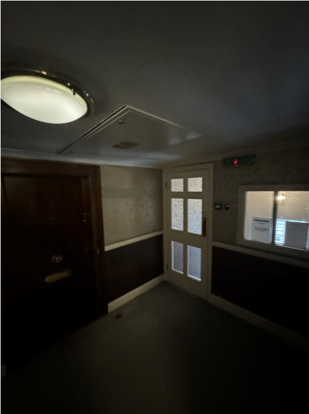
Photograph 9 – Timber stud wall at fourth floor
