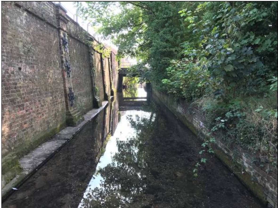
Fig 7 – view south along Beck showing retaining wall of the northeast side
