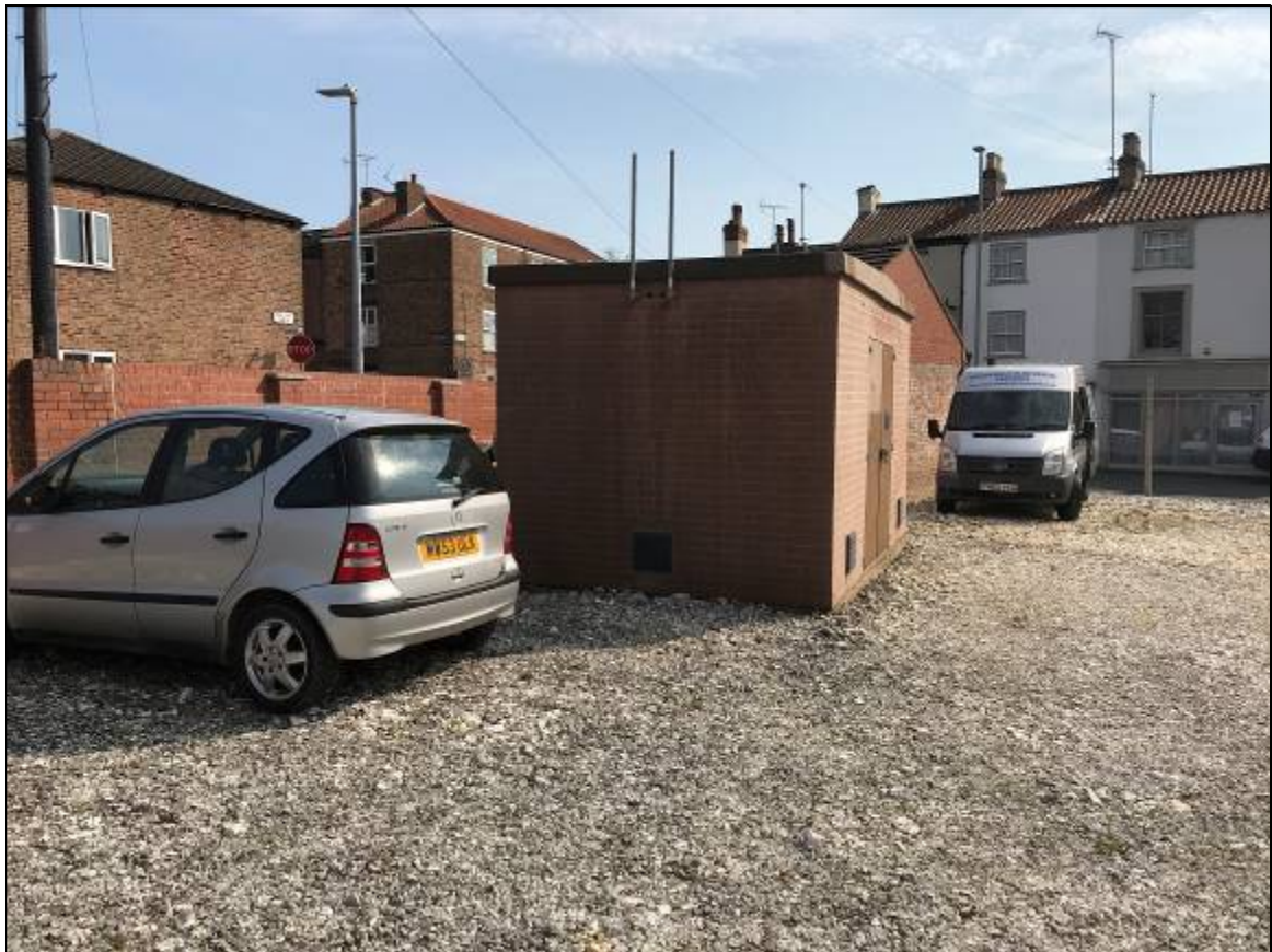
Fig 11 – new gas governor building
