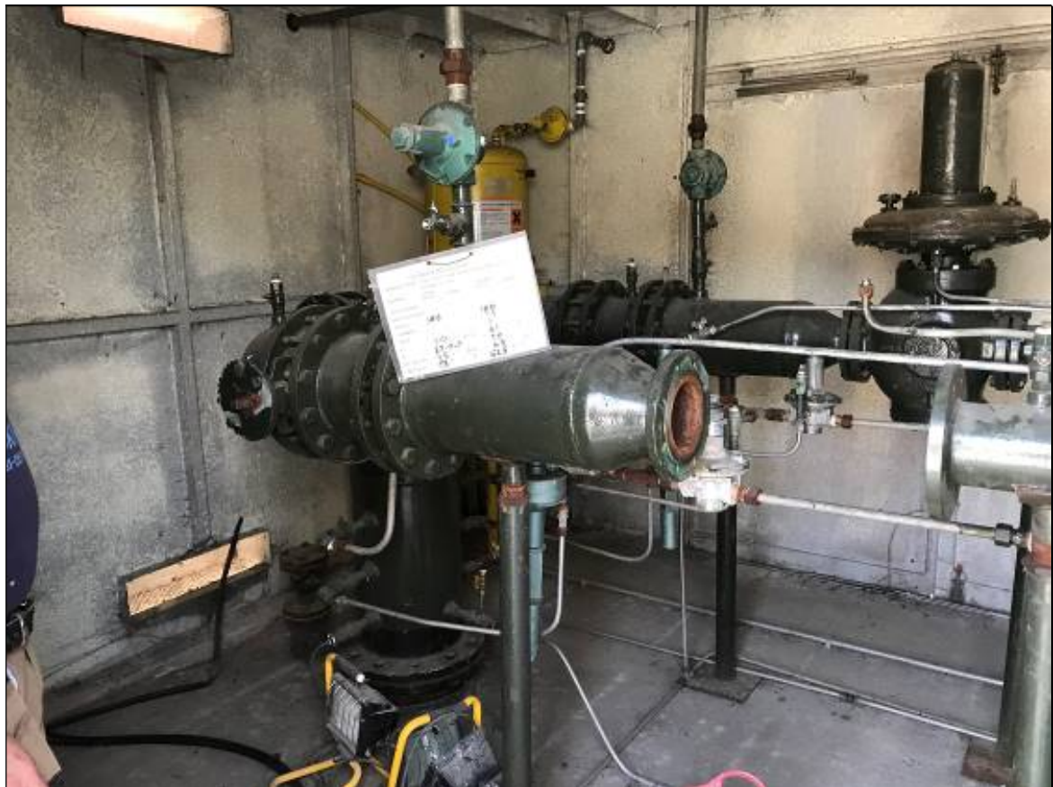
Fig 12 – interior of old gas governor building
