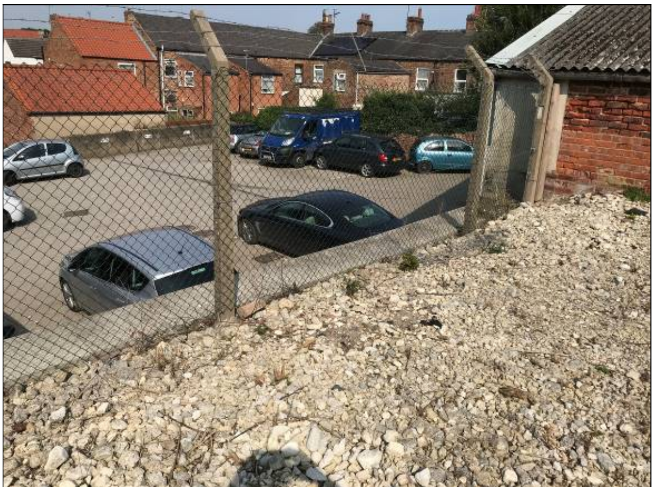
Fig 10 – view to northwest showing drop in level to neighbouring site
