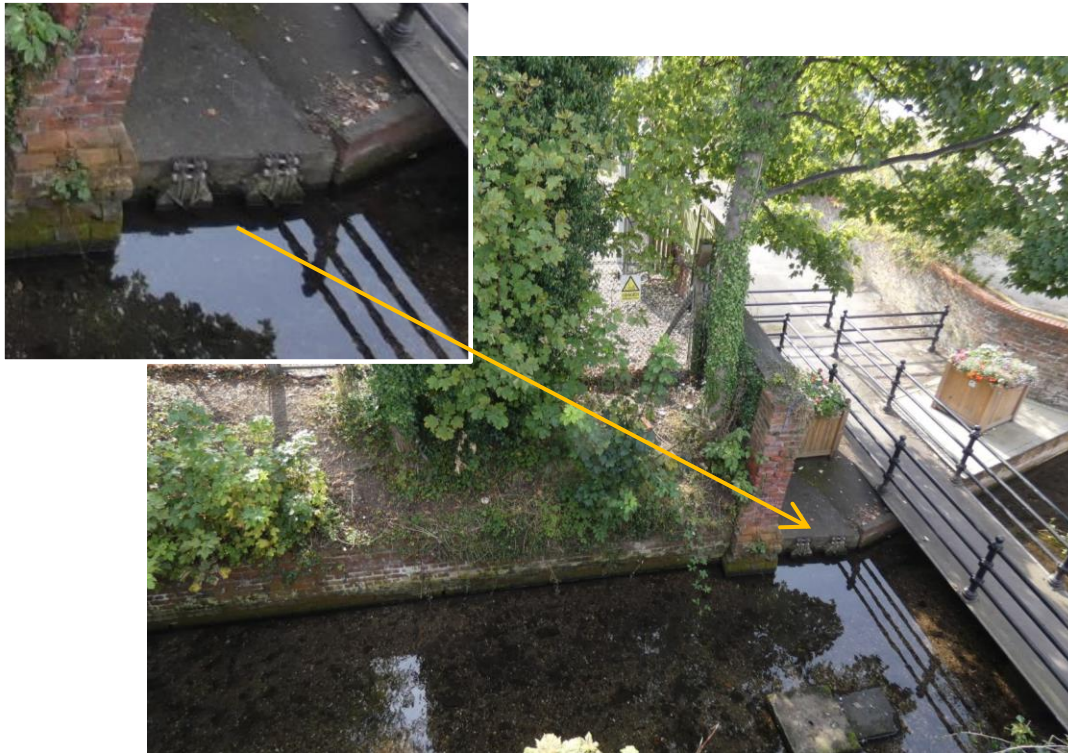
Figure 11.1b – Photo showing the Drifffield Beck & existing YW twin outfalls.
