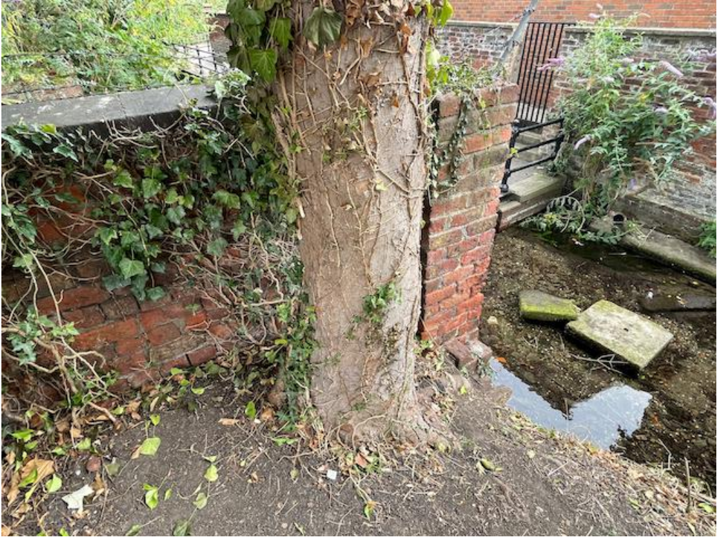
Figure 2. T373 located close to the boundary wall.
