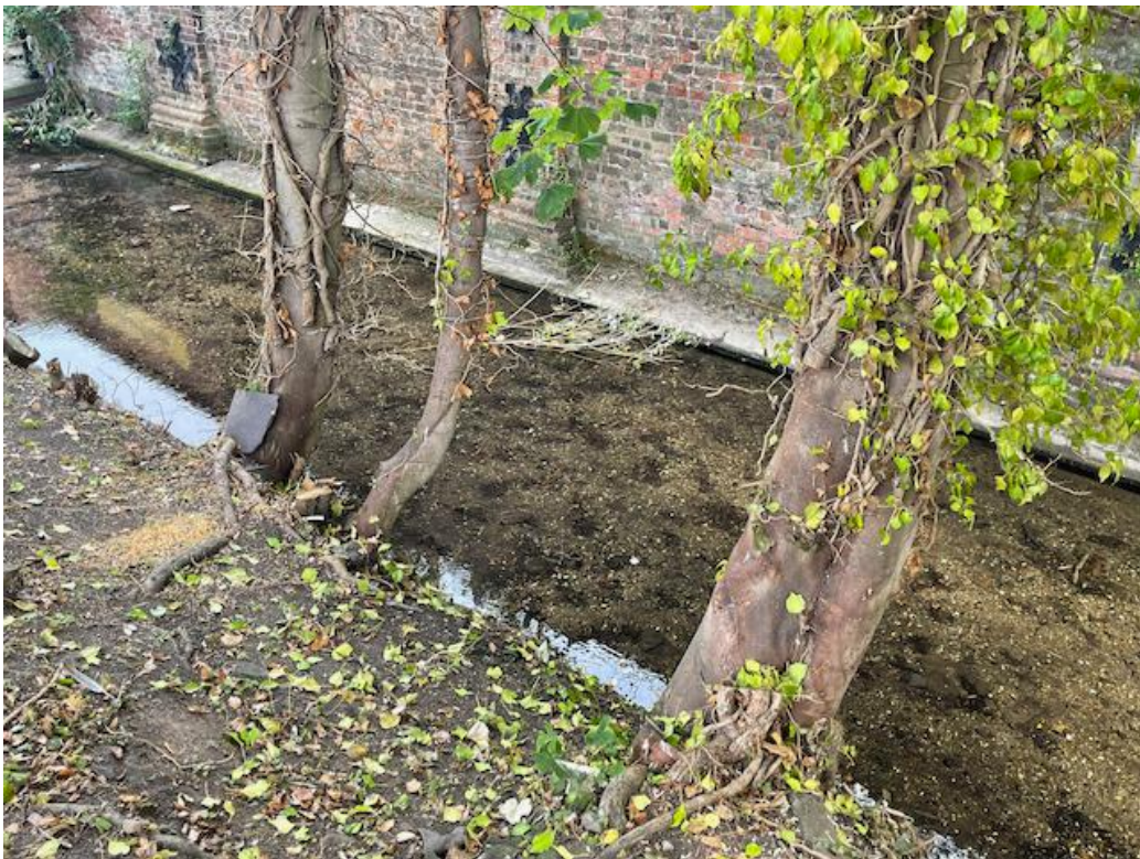
Figure 4. G377 (left) and T378 (right) both located onto of the brick retaining wall.
