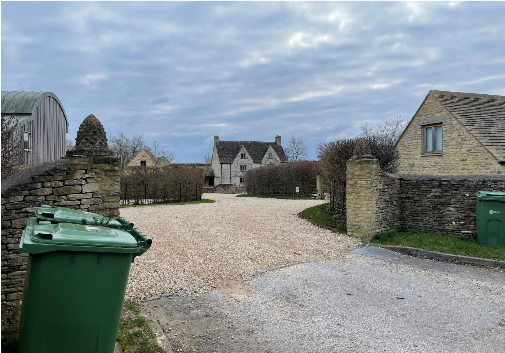
Plate 20: Public south-south-west-facing view of Mill Farmhouse from the main road to the north.
