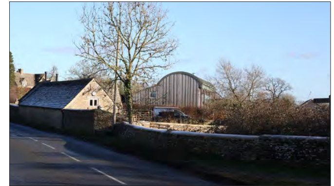
LLCA2-02 Building form and vegetation breaking up elevations
