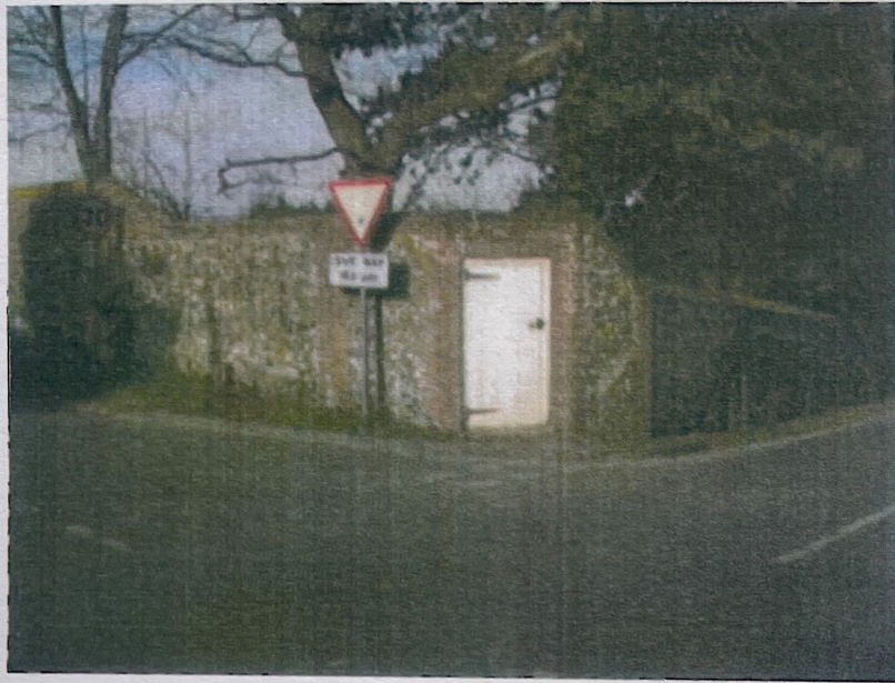
Photo 1- Existing pedestrian gate
