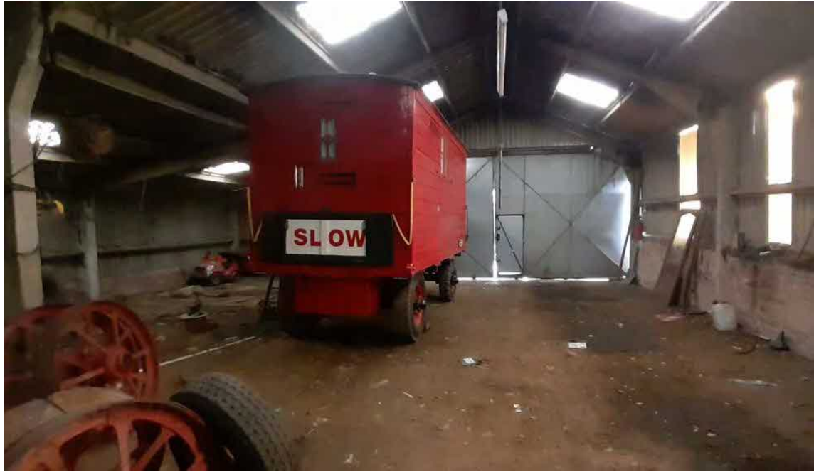
Inside the main shed / garage
