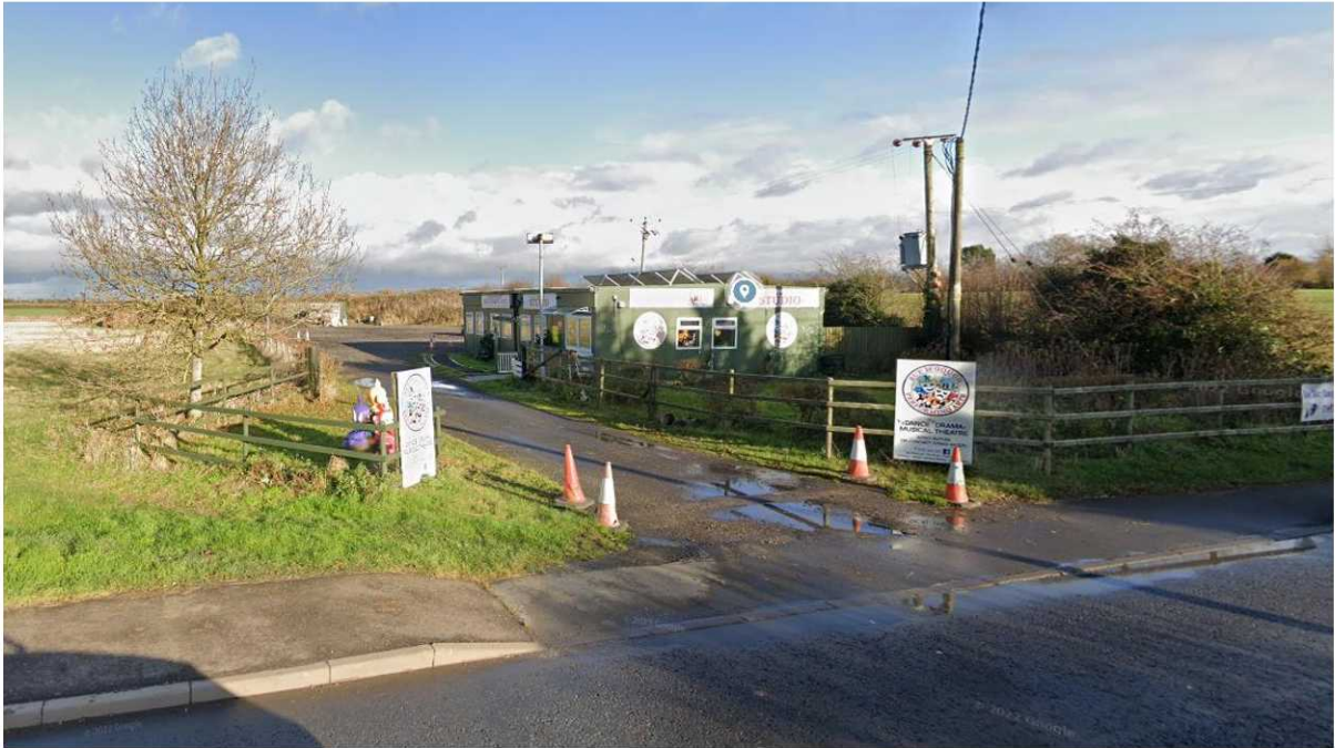
Figure 2: The site viewed from West End looking to the northeast.
