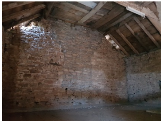
Photo 12: Area above mezzanine floor
