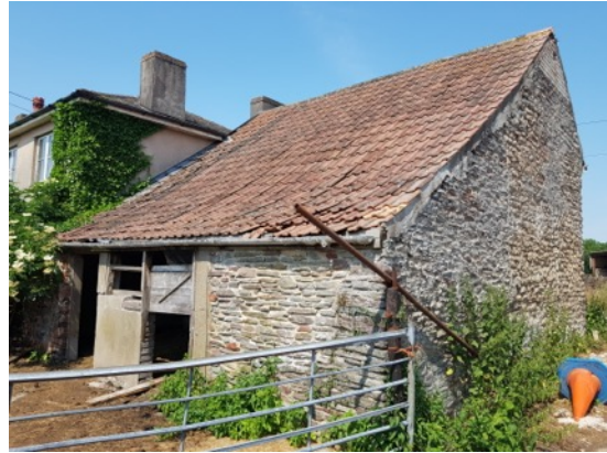
Photo 2: Building viewed from the east
