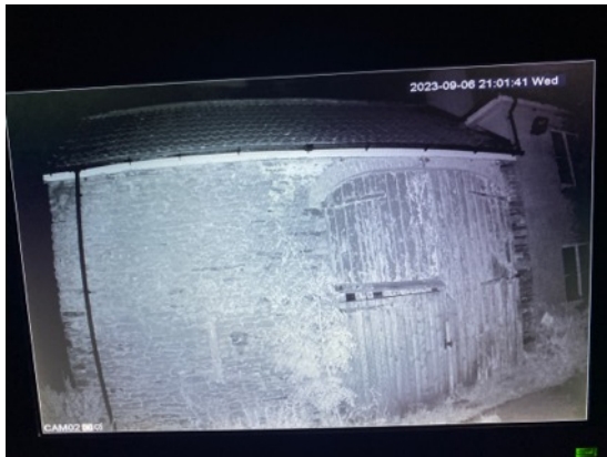
Photo 13: Example infrared camera view – front NW facing elevation.
