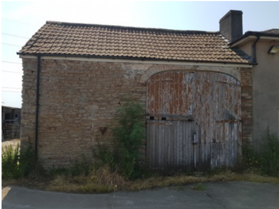
Photo 3: Front, north-west facing elevation
