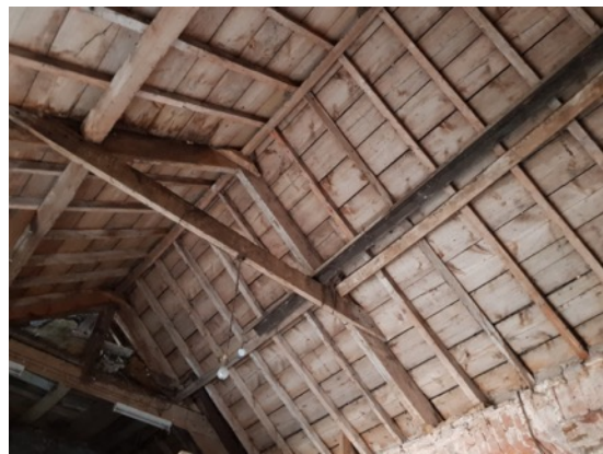
Photo 10: Exposed internal roof structure with wooden boards to underside of tiles
