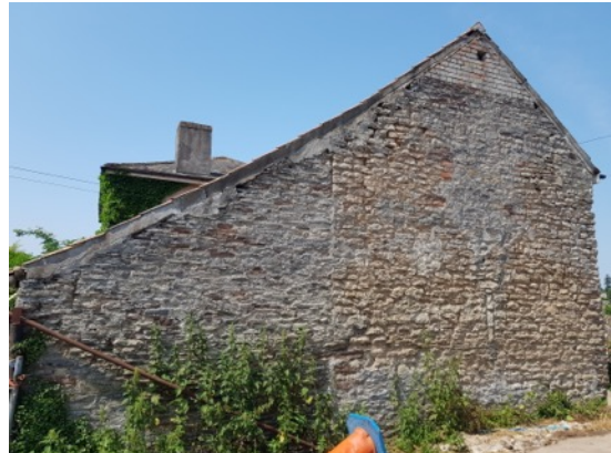
Photo 4: North-east facing gable end wall
