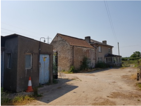
Photo 1: View of building within farm yard with adjoining residential dwelling
