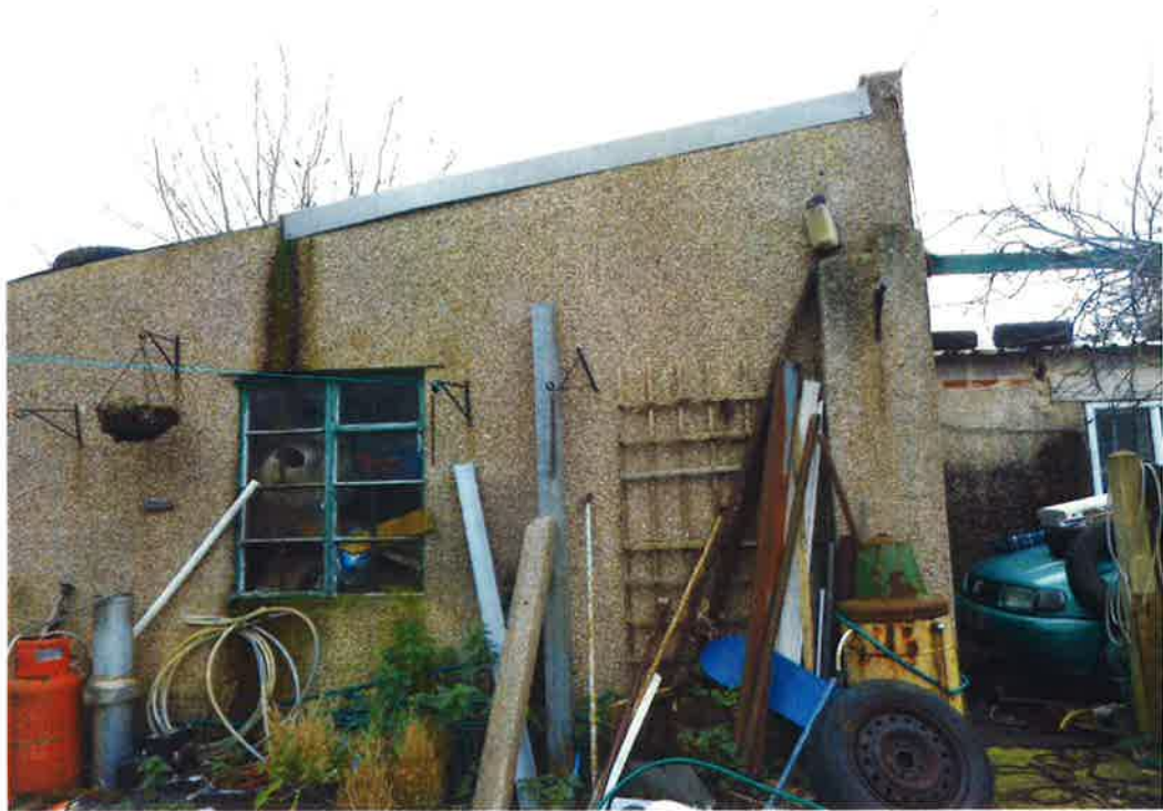
3: North Elevation of Workshop 2
