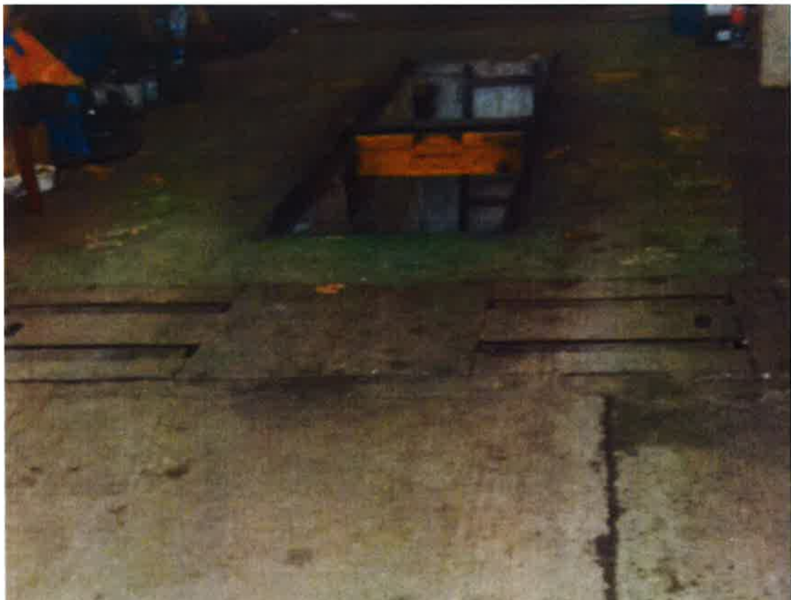
6: Front Workshop Slab and Service Pit
