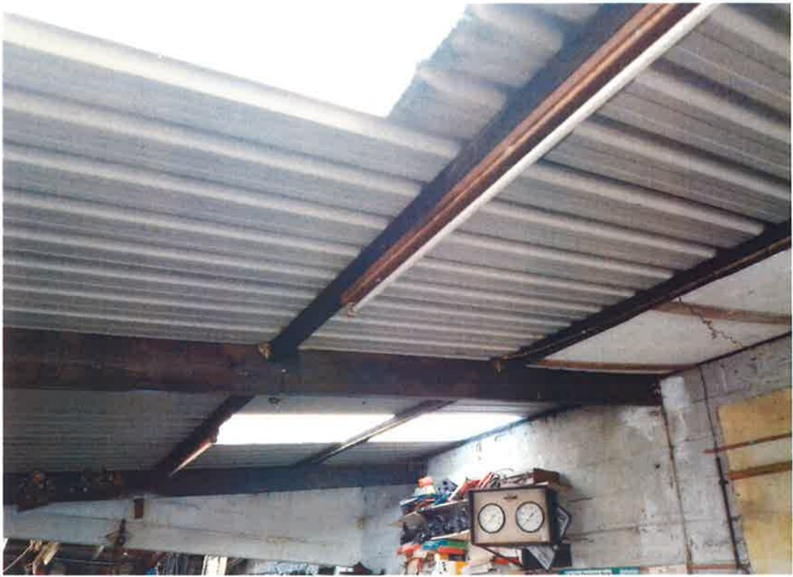
7: Front Workshop Roof Structure
