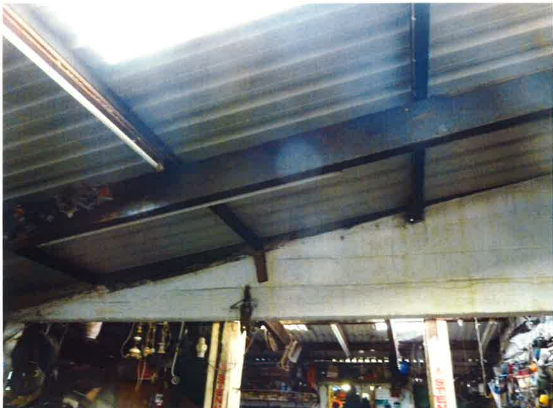
8: Concrete Lintel Between Workshops
