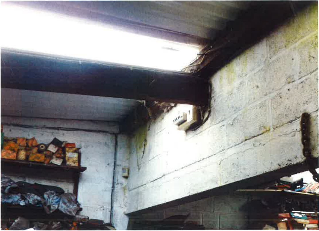
9: Back Workshop Roof Structure
