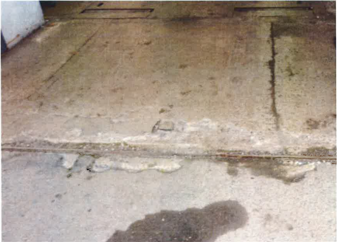
5: Floor Slab at Main Entrance
