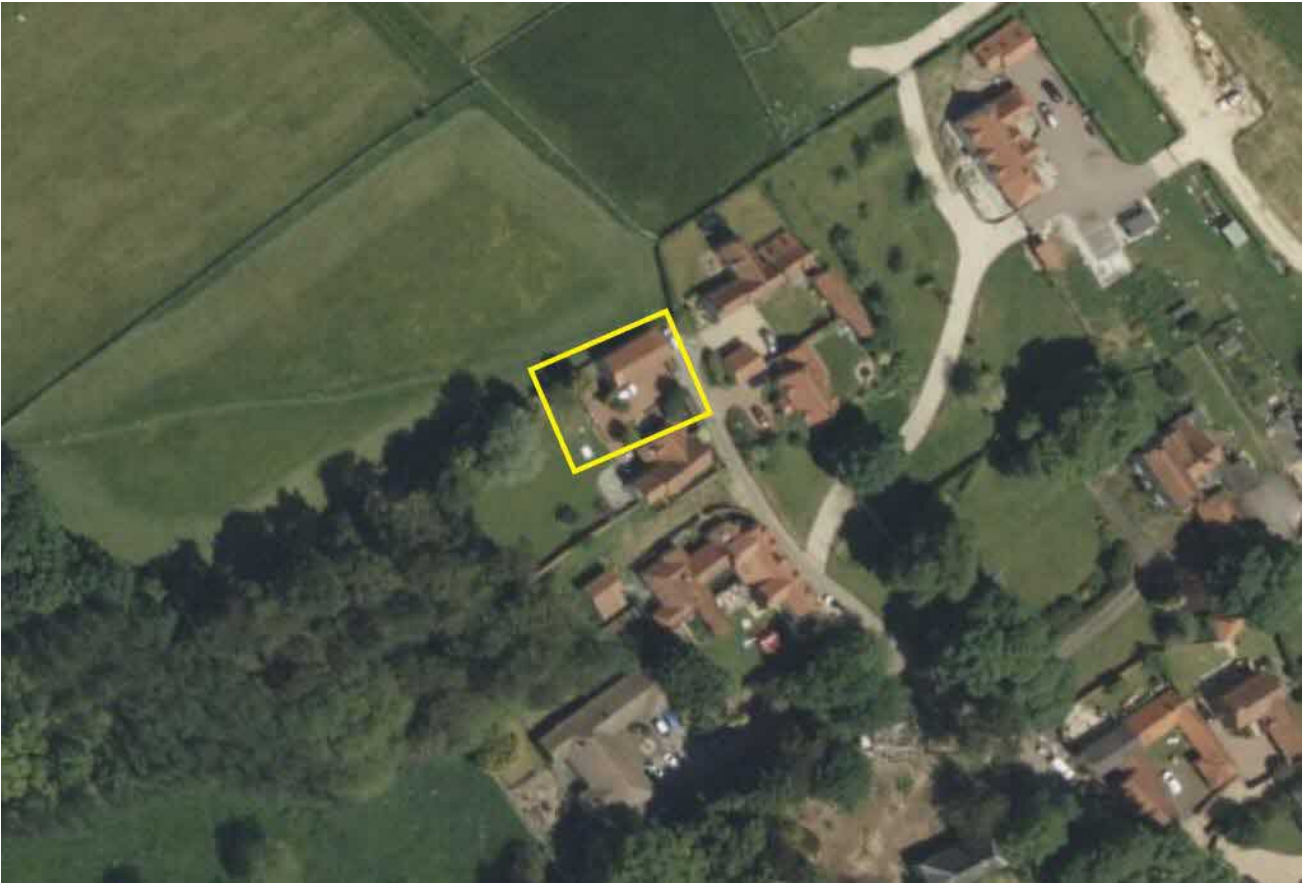
Figure 2: Site Contextual Aerial Photograph
