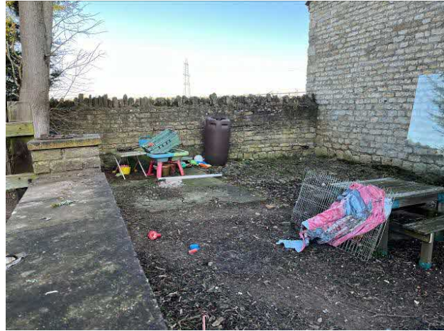
Concrete pad to east side of T4
