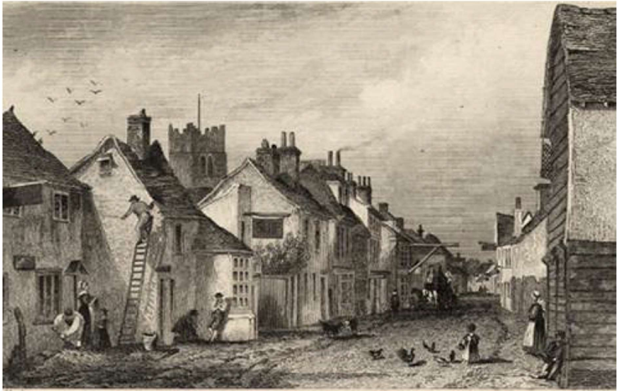
Fig. 2 High Street, Ingatestone, looking south-east towards the Spread Eagle, c.1800 (ERI/LS/COL/00049).
