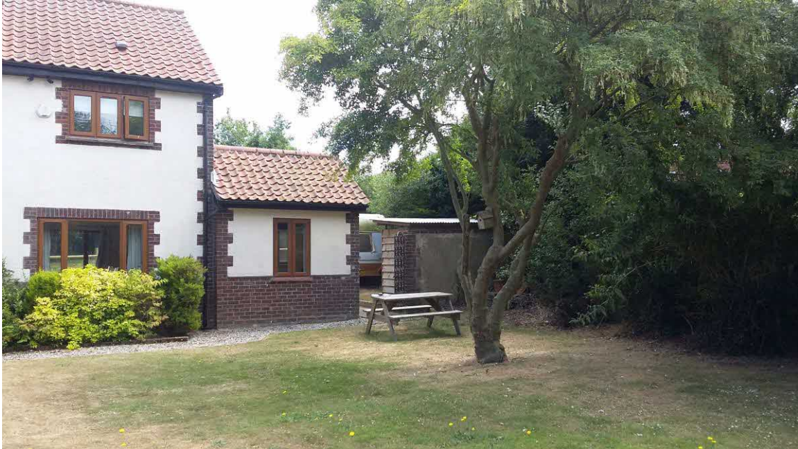
Front view towards southern boundary
