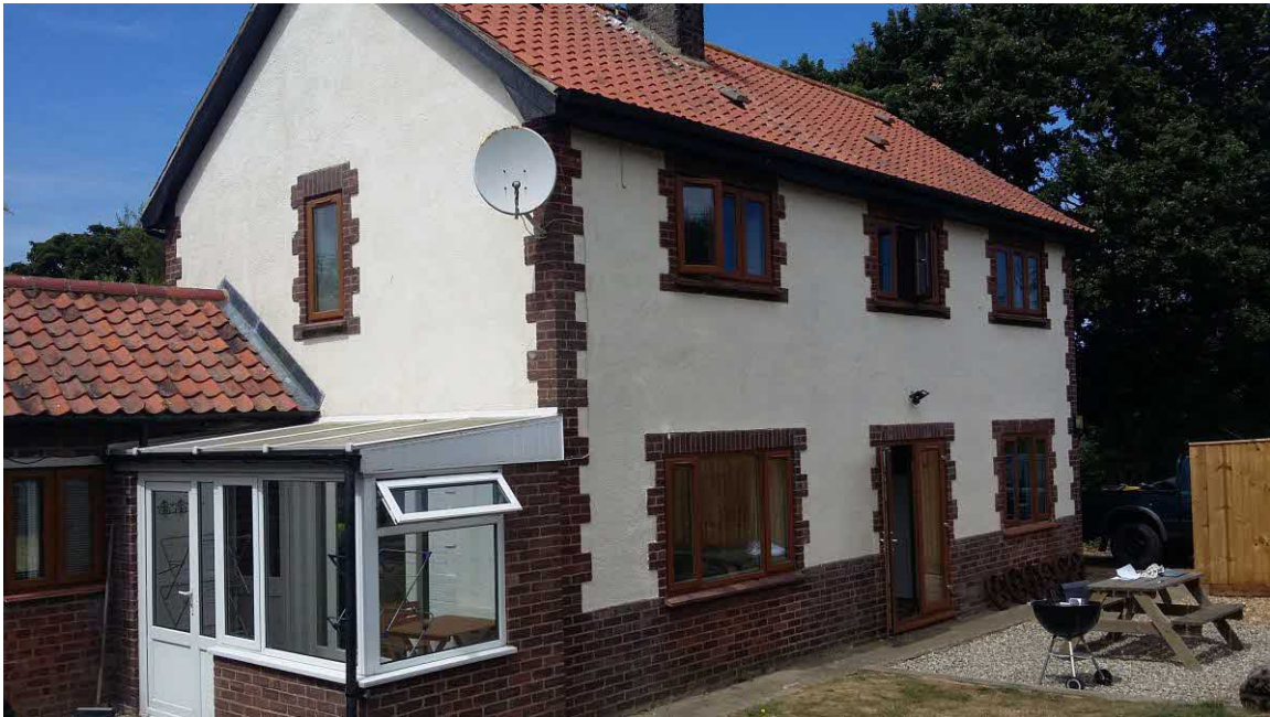
Rear view, existing lean-to conservatory to be removed
