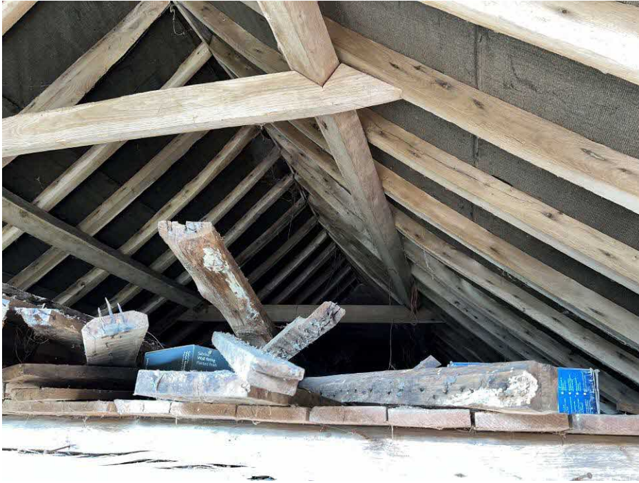
Plate 1 – Internal View of Roof Structure
