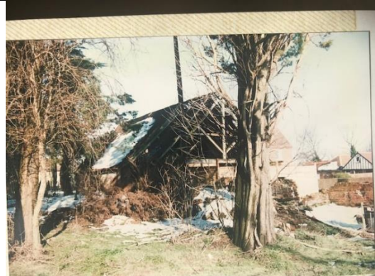
Fig 2. Similar date to photo 1 taken from the south. Note tile roof and largely collapsed southern part of barn.
