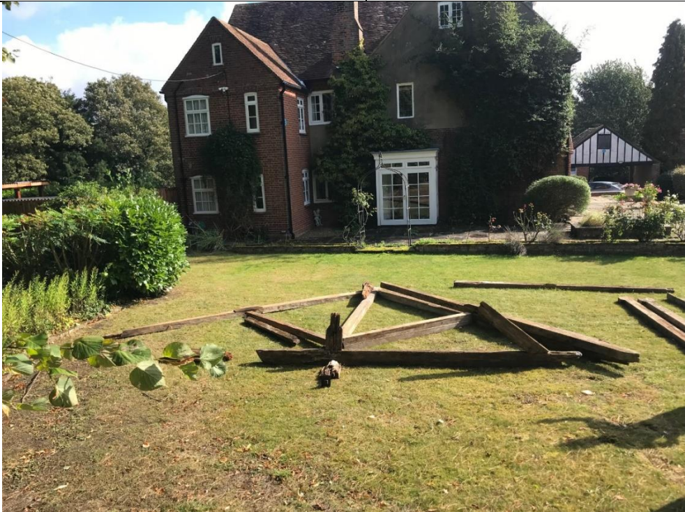
Fig 12. Surviving roof timbers pieced together to form an original truss. This will be reused and replicas created in timber for the remaining trusses.
