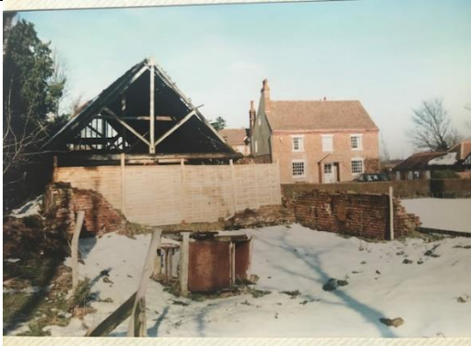
Fig 1. Undated photo of northern part of barn, likely to be 1980s after fire. Note that 3 no. king post trusses appear in the northern part of the barn and the northern gable supported on vertical posts (also seen in Fig 3). At the time of the photo, and the revised list entry, the southern end had collapsed so originally there were 4 bays. Therefore, the evidence shows the roof originally had 3 internal king post trusses with 2 gable ends supported on vertical posts.
