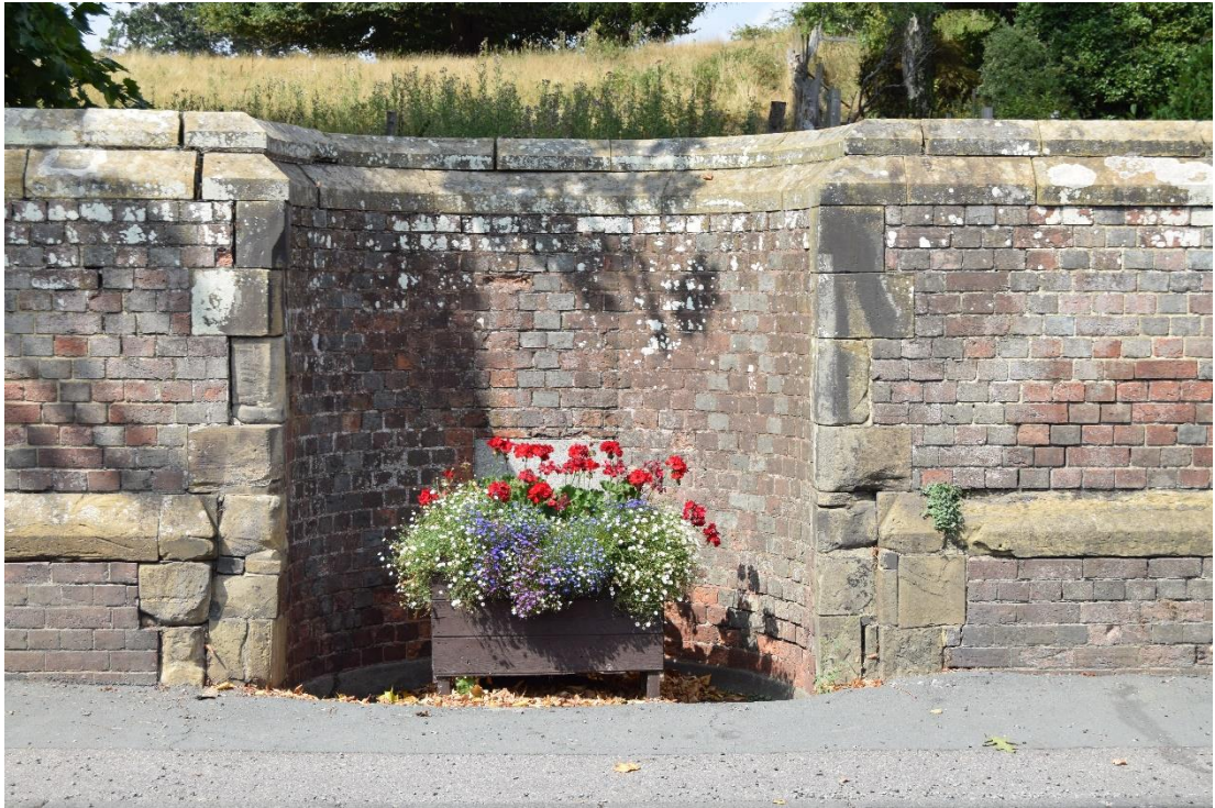
Plate: Section of park wall facing High Street
