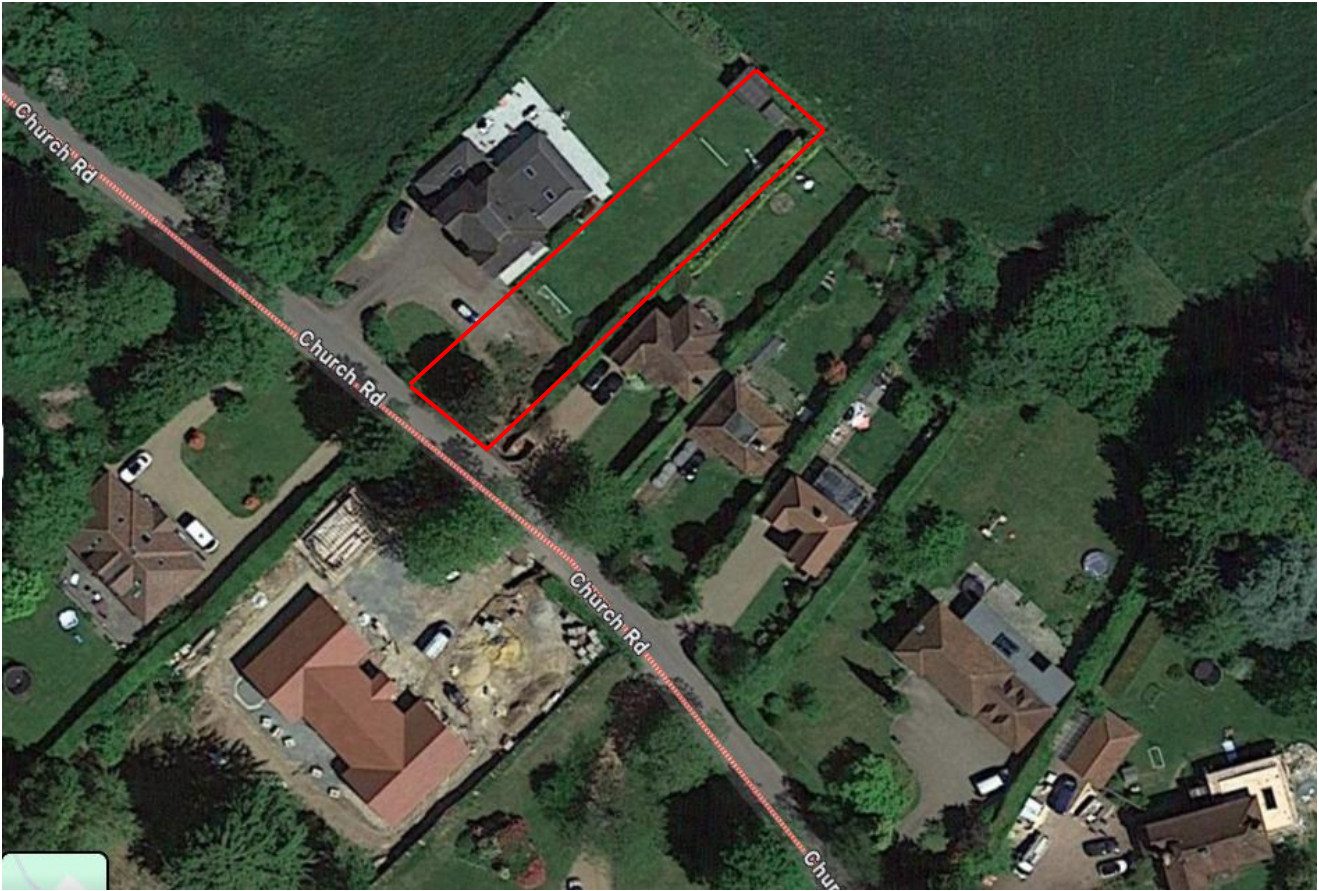
Aerial view of the application site
