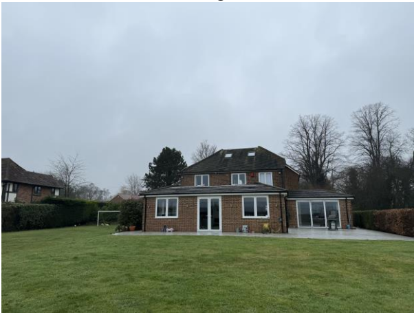
▲ Fig 4. Photo showing the back of the existing house
