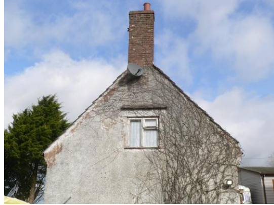
South facing end.
