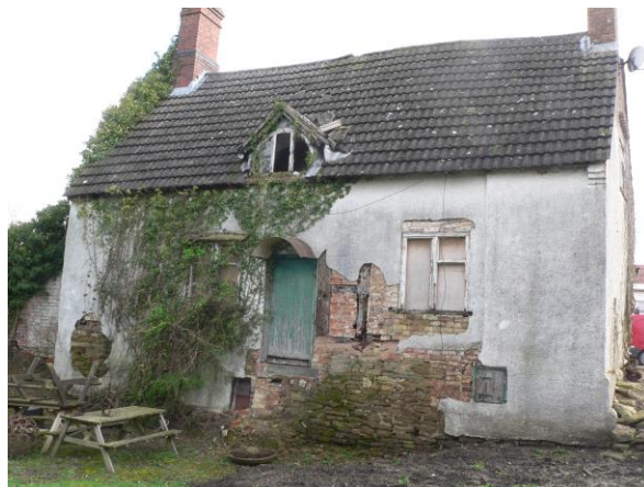
Front view (west facing)
