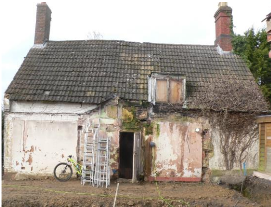
Rear view (east facing)
