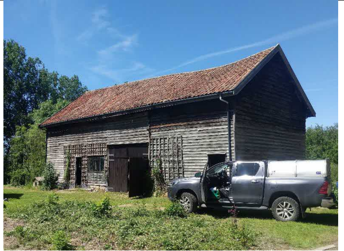
Photo 2 South and west elevations
