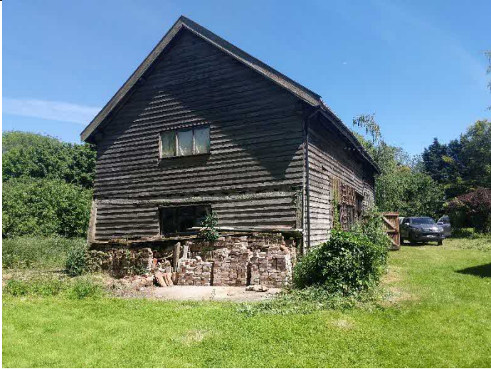
Photo 1 West and south elevations
