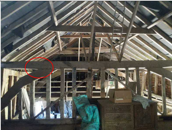
Photo 11 Internal view of the barn – tiebeam/brace where Natterer's are roosting
