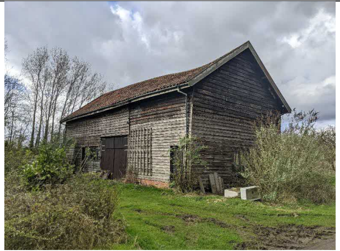
Photo 14 Barn south and east elevations
