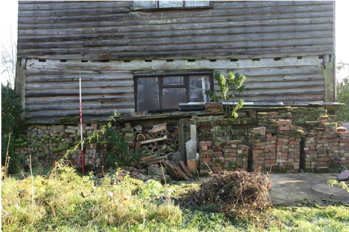
Illus. 3. The western external gable showing its modern glazed windows and renewed cladding with a full complement of joist mortices in its chamfered binding joist for the ceiling of a demolished bay that extended into the foreground. The joints have diminished shoulders as found in high-quality carpentry of the mid-16 th century and later (as shown in illus. 20). Pegged mortices for projecting mid-rails are also visible in the present corner posts.
