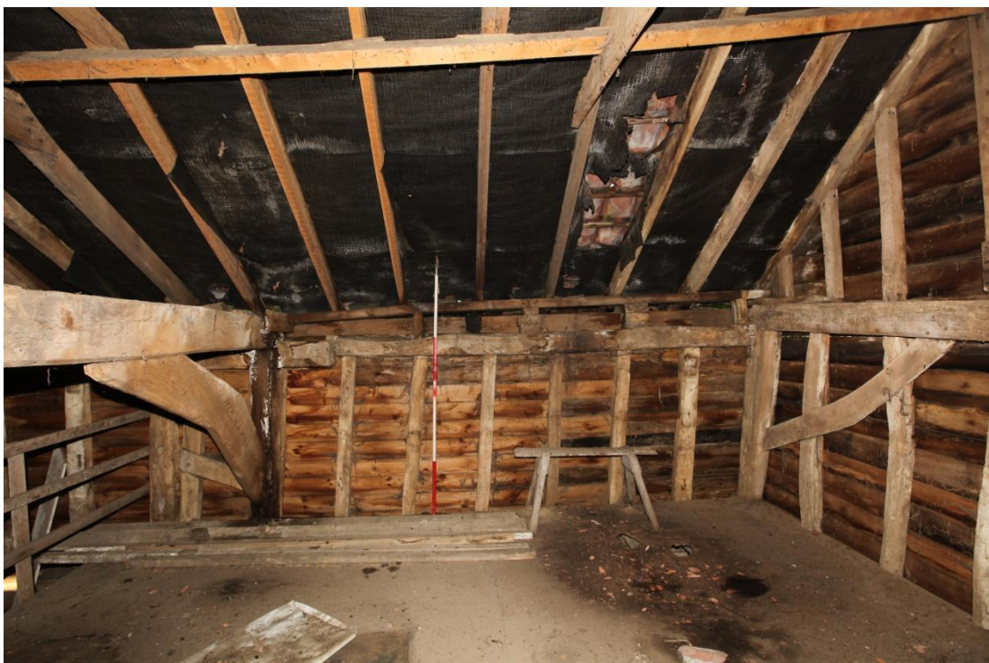
Illus. 10. The northern internal wall of the eastern bay's loft (D) which retains its original narrow studs with a trench for a missing corner brace on the right. A crude scarf joint links the roof-plate to the earlier plate of bay C on the left (see illus. 11).
