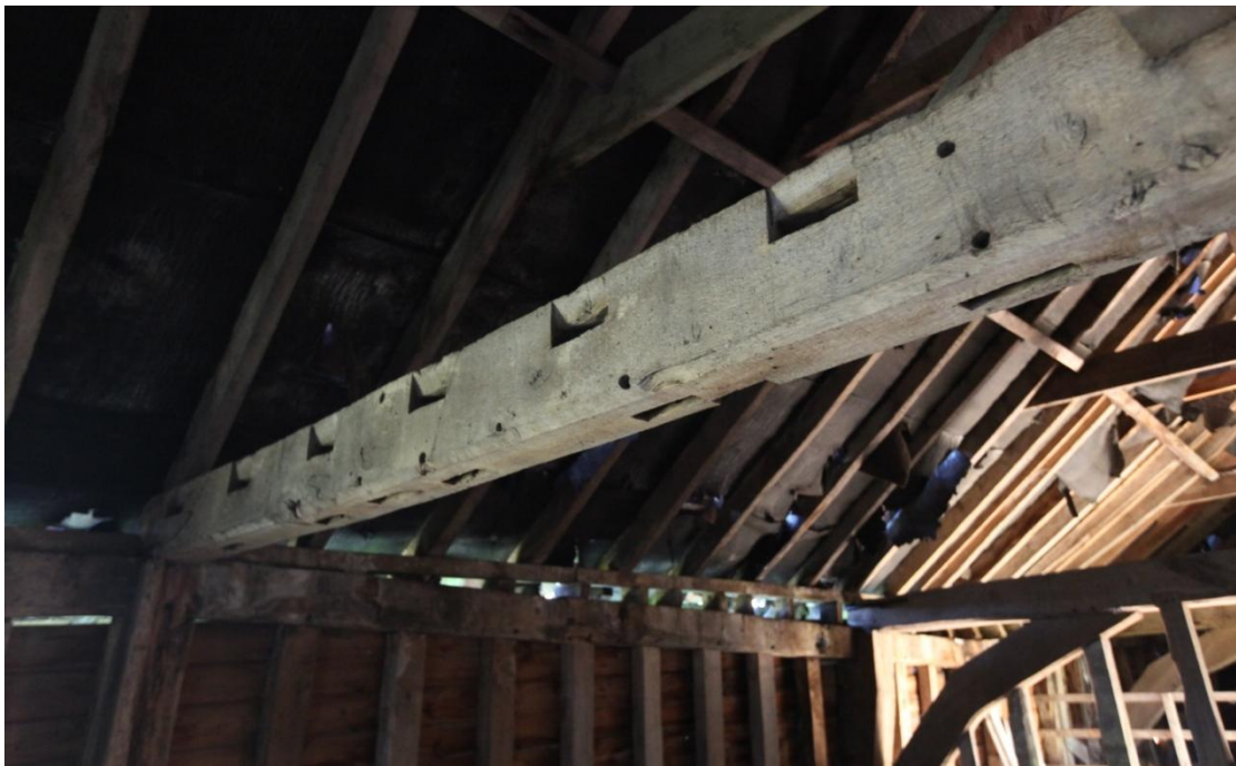
Illus. 20. The western face of the tie-beam between the floored bay (A) to the left and the three-bay threshing barn in bays B-D showing its neat chamfer and pegged stud mortices for a missing solid partition. The joist mortices held soffit tenons with diminished shoulders in a style normally found only in high-quality domestic ceilings between the mid-16 th and mid-17 th century when tall sectioned joists became the norm.
