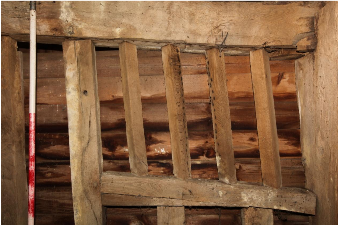
Illus. 23. A detail of the intact first-floor window in the southern wall of the westernmost bay (A) with the 12-inch wide storey post that now forms the corner of the truncated building to the right. The original diamond mullions are uncommon survivals even in normal domestic contexts and are rare in barns. The nails flanking the central light are usually found in conjunction with leaded panels of glass and could be explained by the insertion of such a panel here when the rest of the window was blocked.
