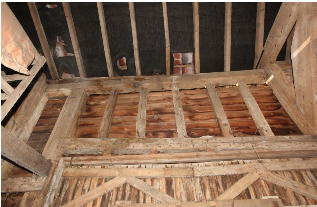
Illus. 6. The southern roof-plate of the threshing bay (C) showing inserted re-used studs above the present door lintel (nailed rather than pegged to the plate). The circular holes at both ends secured the pin hinges of the original doors in a manner rarely seen in south Suffolk where iron hinges were the norm. The jamb post on the left was thought necessary to stabilise the corner post which abutted an earlier structure.
