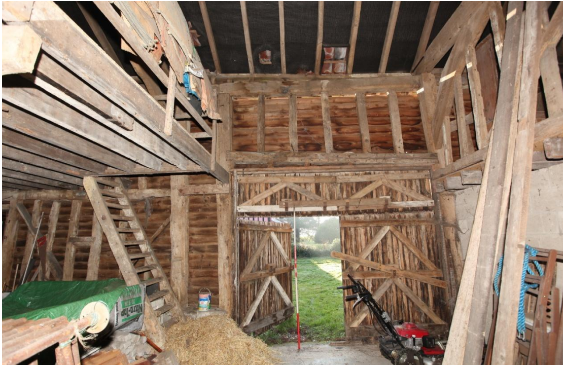
Illus. 5. The southern interior of the threshing bay (C), now with a modern concrete floor and 20 th century storage lofts of tall-sectioned softwood joists on both sides. The original doors rose to the roof-plate but unusually were defined by a single large post 18 inches to the right of the bay's arch-braced storey post on the left. The eastern loft in bay D on the left projects into the bay by the same extent.
