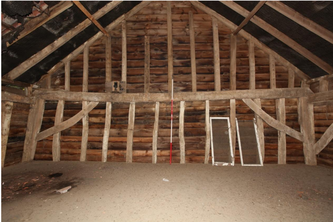
Illus. 9. The eastern internal gable from the 20 th century loft in bay D. The framing of this bay is very different to that of bays A-C with much narrower and more widely spaced studs. It dates from the 17 th century and evidently replaced an older structure against which bay C was originally built in the late-16 th century. The lower and most of the studs above are pegged to the tie-beam and original to the fabric, as are the internally trussed corner braces.
