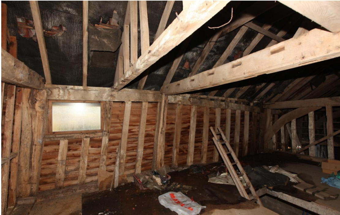
Illus. 17. The northern internal wall on the loft in bays A and B showing the position of an original first-floor window occupied by the modern glazed window to the left (with a detail in illus. 18 below). The tie-beam that divides the two bays on the right contains empty pegged mortices for a missing solid wall against the threshing barn in bays B-D and joist mortices for a missing first-floor ceiling in bay A.
