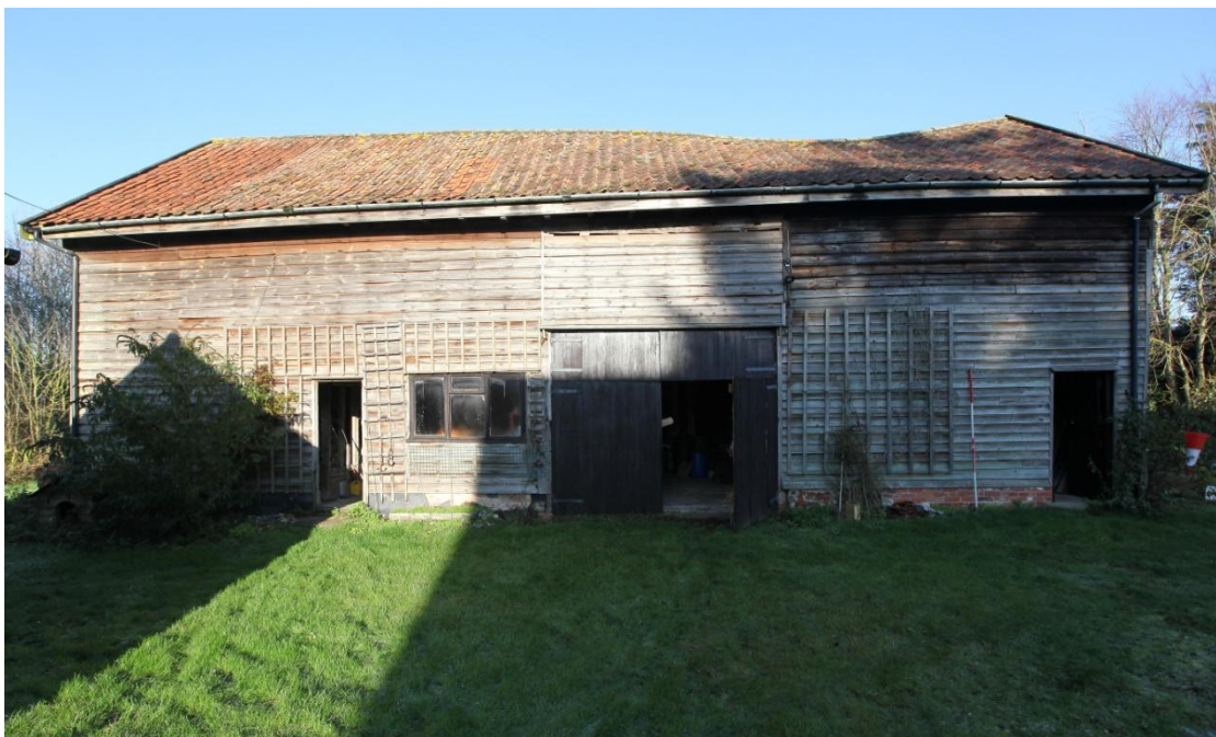
Illus. 4. The southern facade of the barn (1) showing its pantiled roof and late-20 th century weatherboarding with a small section of tarred weatherboarding to the loft in bay D on the right that may survive from the late-19 th or early-20 th century refurbishment. The outline of the original full-height doors to the main entrance in bay C is visible above the present double doors of the late-20 th century.
