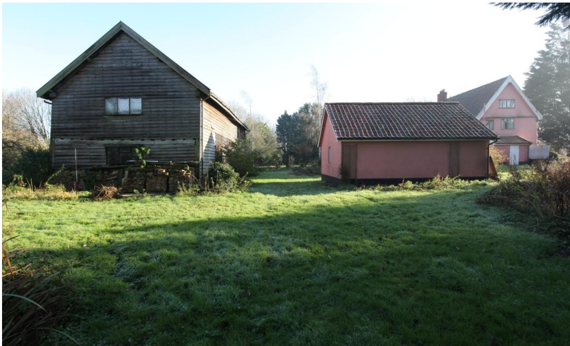
Illus. 2. A view of the site from the west showing the modern garage (2) between the barn (1) on the left and the grade II-listed house (3) in the rear to the right. The barn’s low-pitched pantiled roof is a late-19 th or early-20 th century replacement of the original, which would have been steeply pitched like that of the house for peg-tiles or thatch. Until its truncation in the mid-20 th century the barn continued into the foreground, stopping just short of the pond visible at bottom left.
