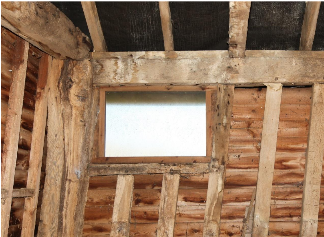
Illus. 18. The original first-floor window in the northern wall of the westernmost bay (A) which retains its original pegged sill with a narrow groove in the roof-plate for a shutter sliding to the right and four empty mortices for missing diamond mullions.
