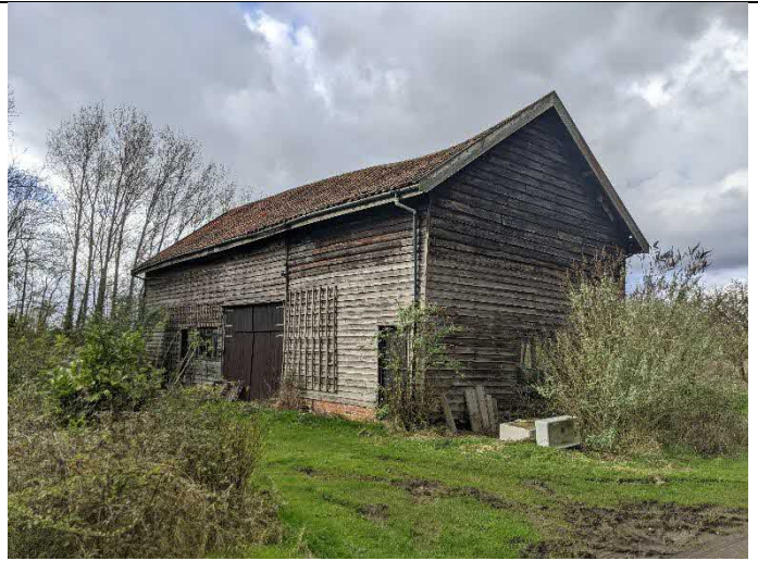
Photo 14 Barn south and east elevations
