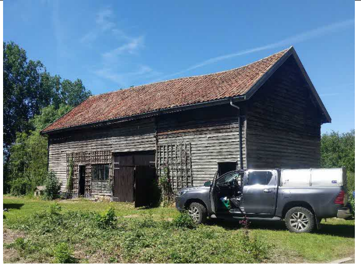
Photo 2 South and west elevations
