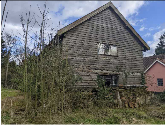
Photo 13 Barn west and north elevations
