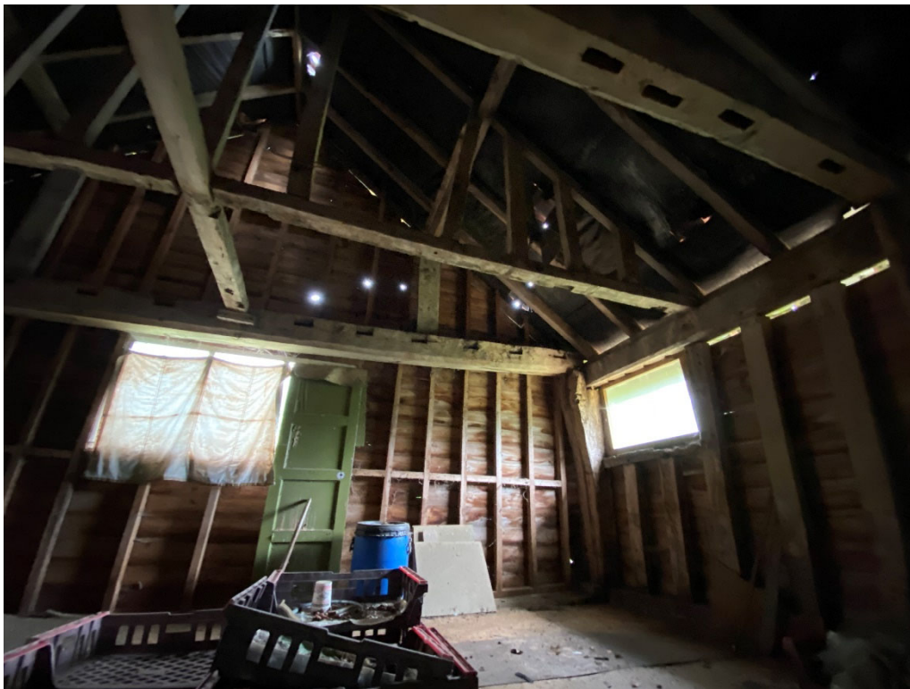
North West First floor with rems of mullion window on right
