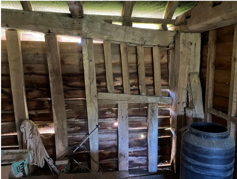
South West Mullion window
