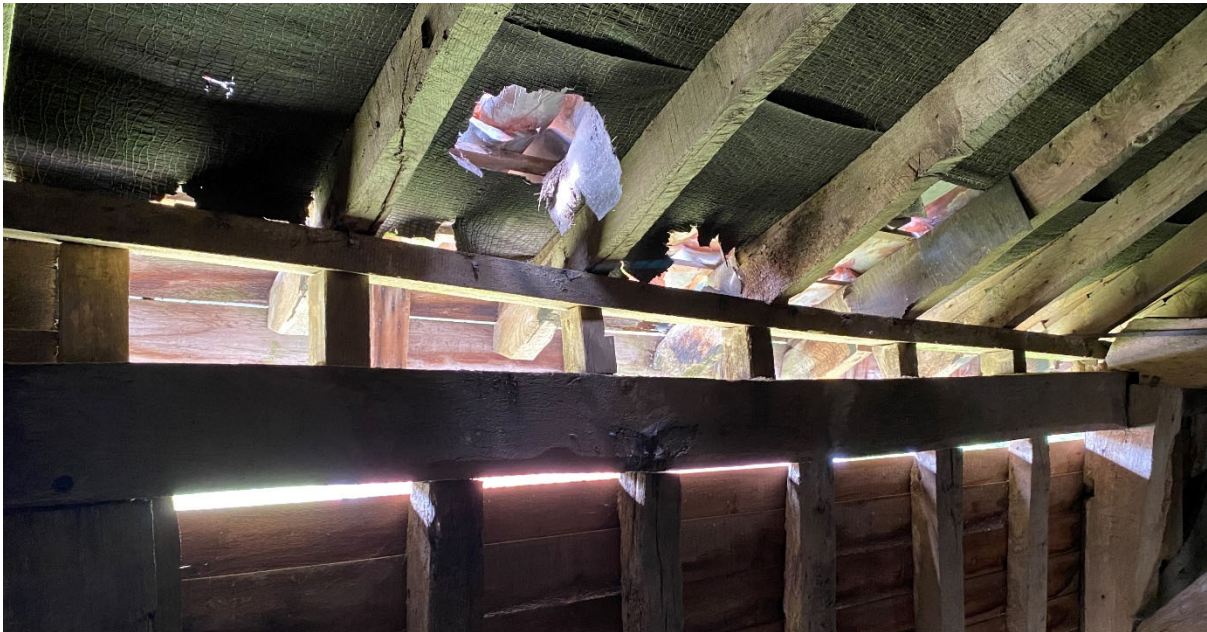
Plate detail showing new wall plate raised on top of existing / levelled in later timber to carry rebuilt roof (above and below)
