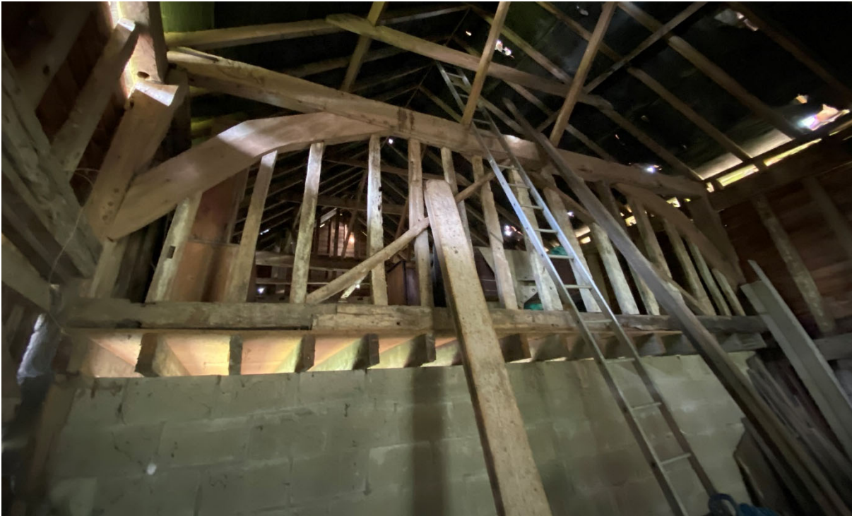
Mainstery looking West – with blockwork (to be removed ) at ground floor
