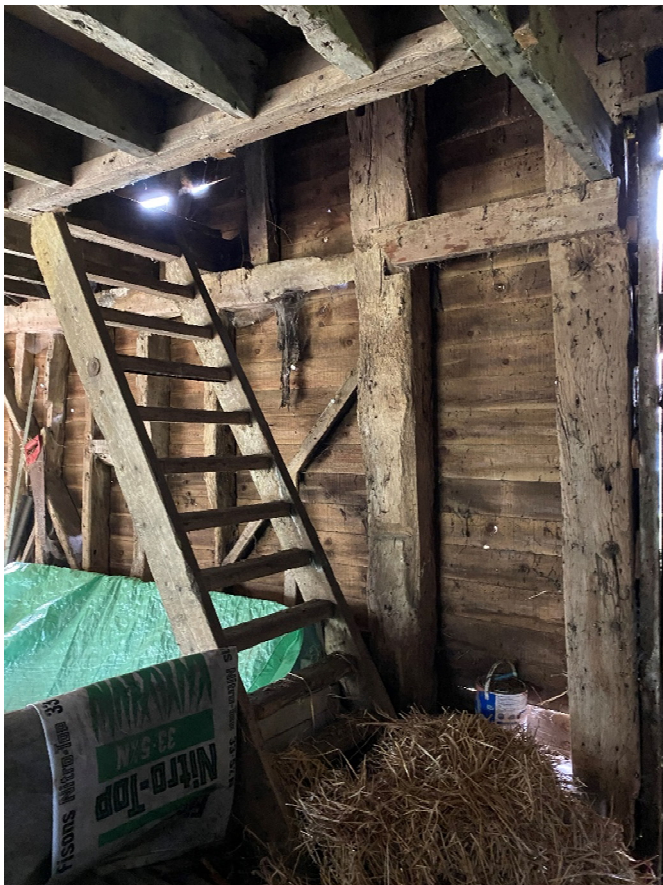
Ladder to East loft
