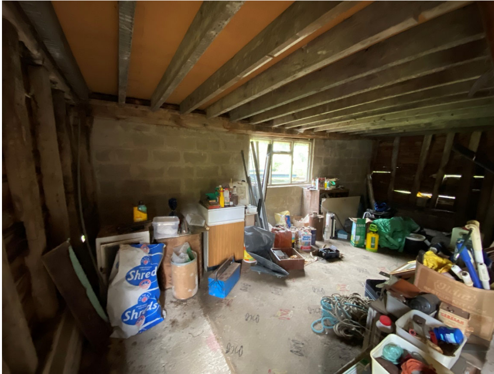
Ground Floor – Western bay – modern block gable wall – to be removed
