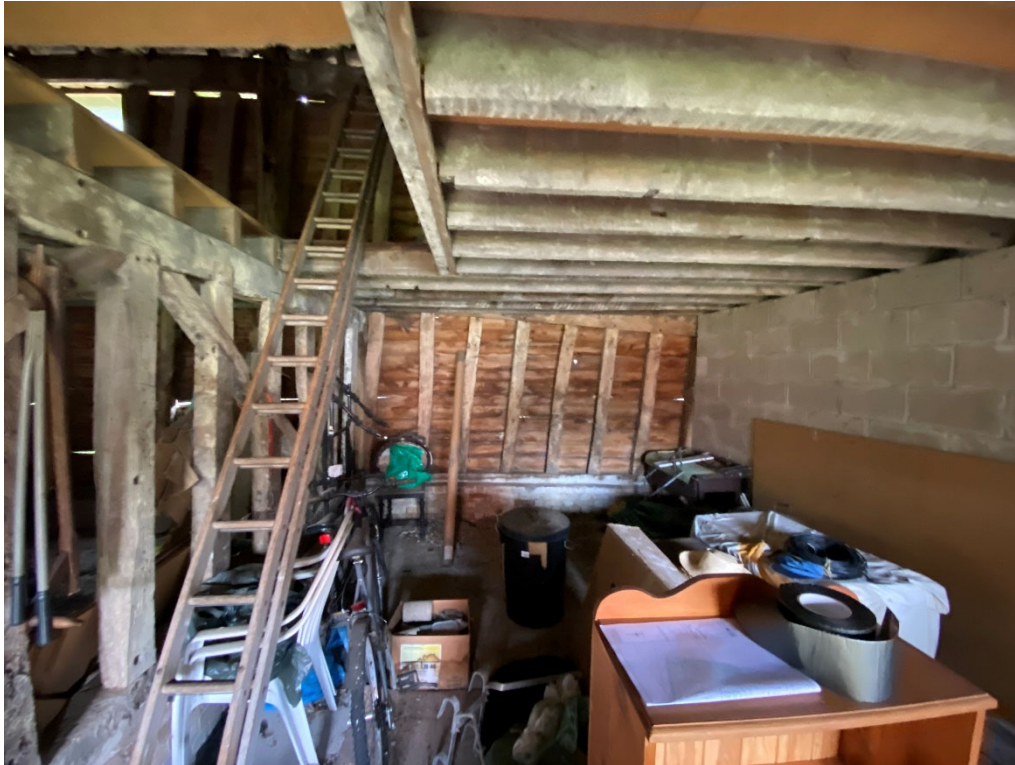
Ladder access through modern floor to West first floor area
