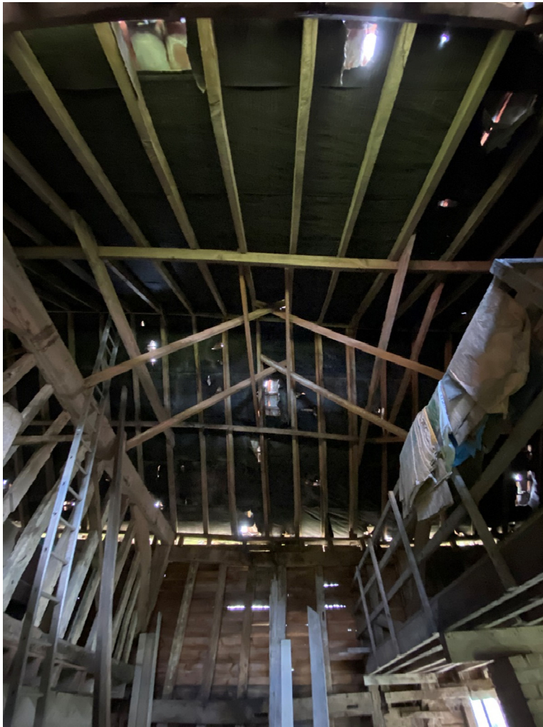
Mainstrey looking North Rebuilt roof and strutting visible
