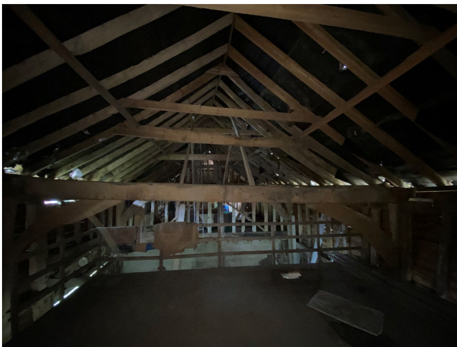
Roof looking West toward Mainstrey
