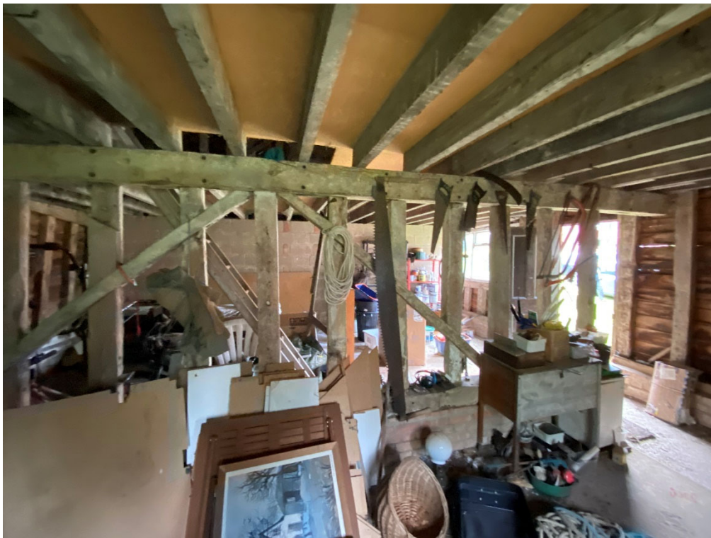
Earlier ground floor stud partition between Western bays
