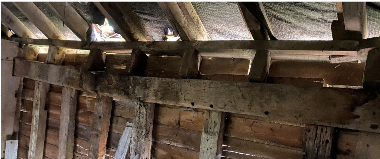
Plate detail showing new wall plate raised on top of existing / levelled in later timber to carry rebuilt roof (above and below)
