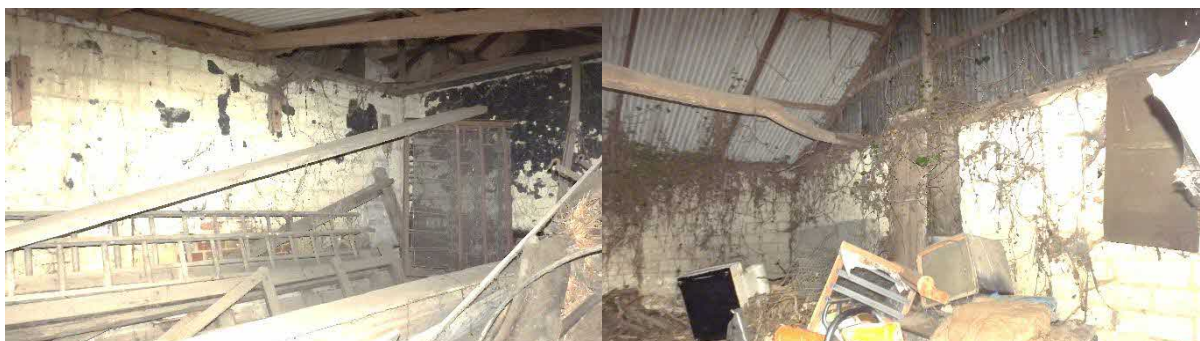
Fig 11 & 12. Internal view of brick, block and clay walls (left) and roof structure (right)
