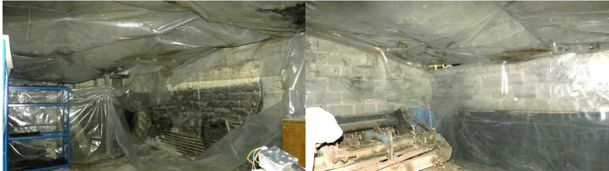
Fig 7 & 8. Well pointed brickwork (left) and roller door access (right)
