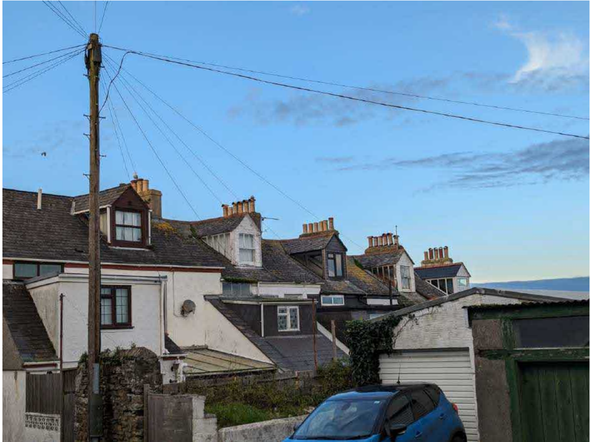
Existing Dormer Extensions on Marlborough Road, Falmouth
