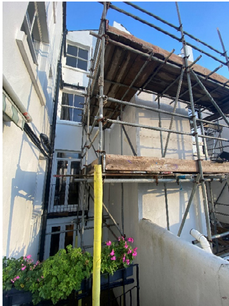
Figure 1, 2, 3 & 4: Existing rear and rear/ side elevations
