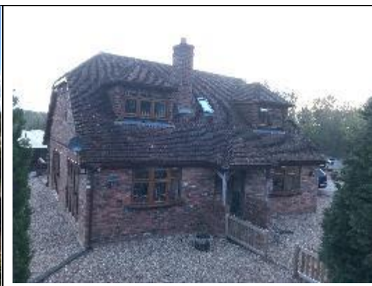
Photograph 2 – South and West aspects
