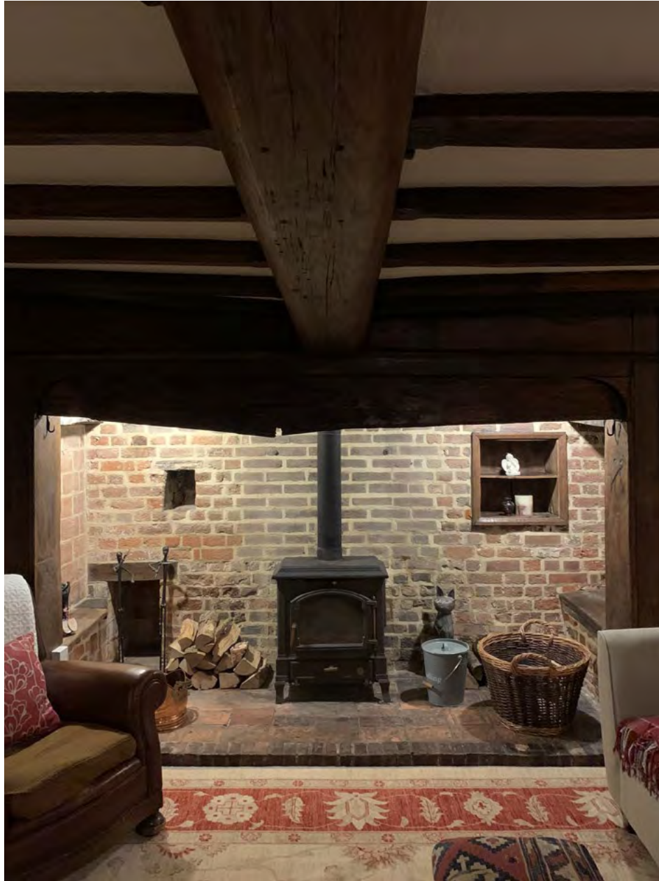
Ceiling joists above the South fireplace
