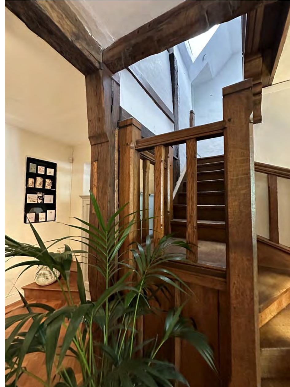
19 th Century timber stair
