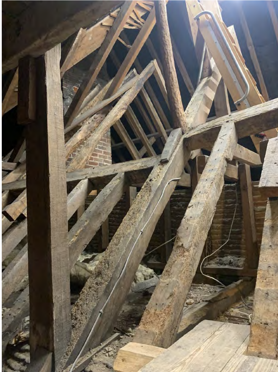
Double roof structure
