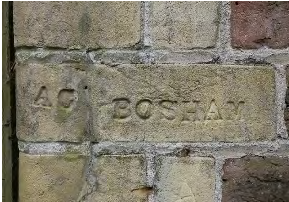
Top - brick hearth at Strange Hall South Above - a brick at Carmelite Convent Chichester, marked AC for Alfred Cheesman
