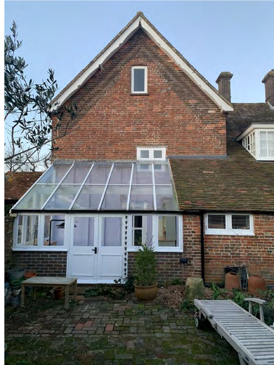
Brick infill to the South facade
