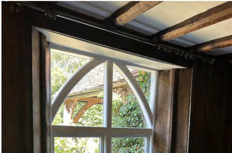
West facade porch and pointed window
