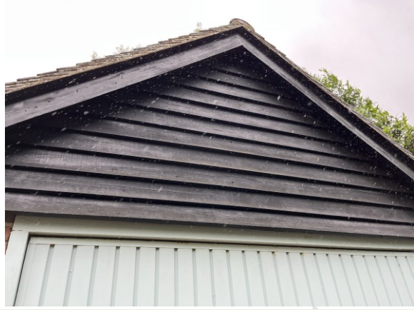
The wooden cladding is tight with no gaps
