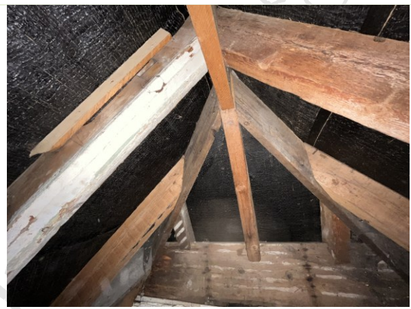
The topmost loft void
