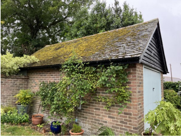
The garage – northwest orientation
