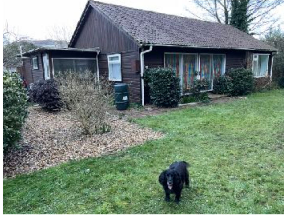
View of principal elevation facing Bedbury Lane.
