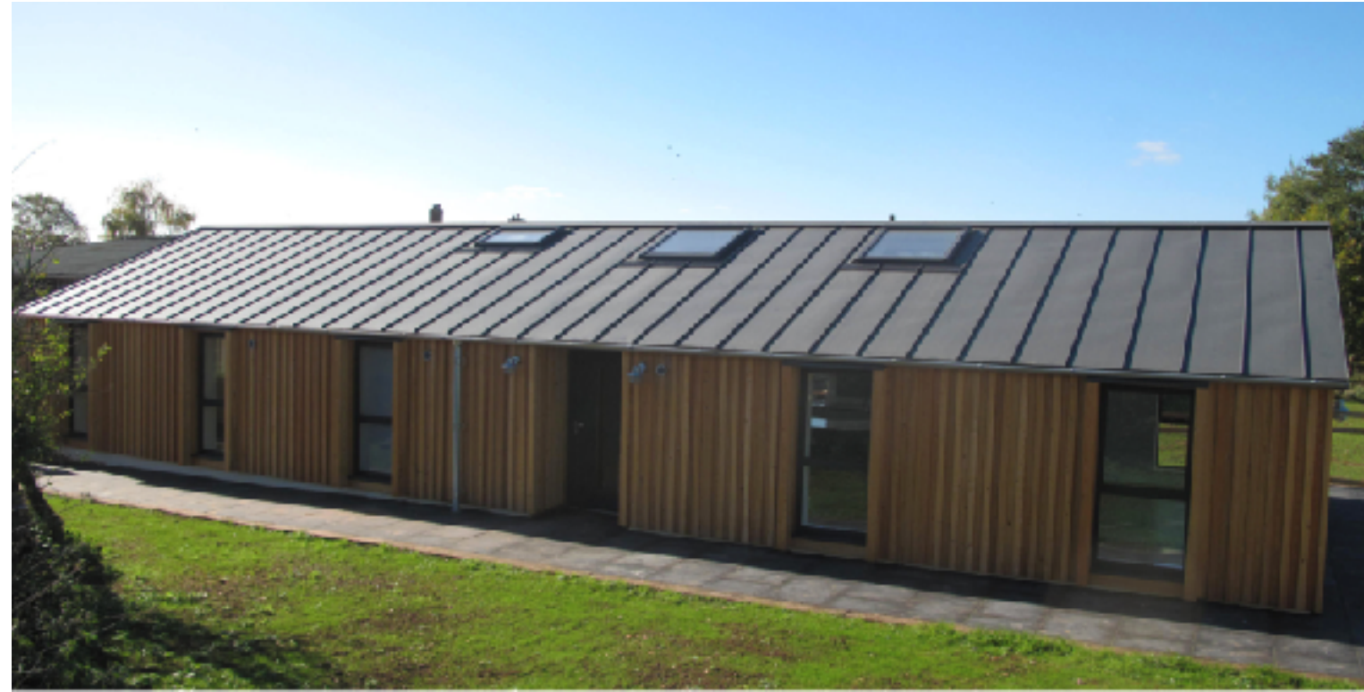
Standing seam zinc roof in light grey.
