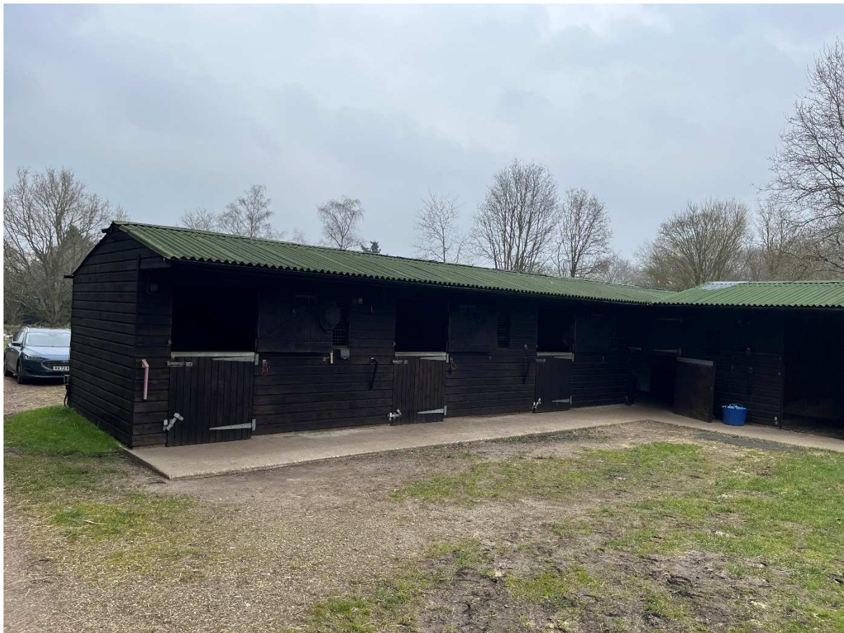
Figure 7. Building C: South Stable southern and western elevations looking northeast.
