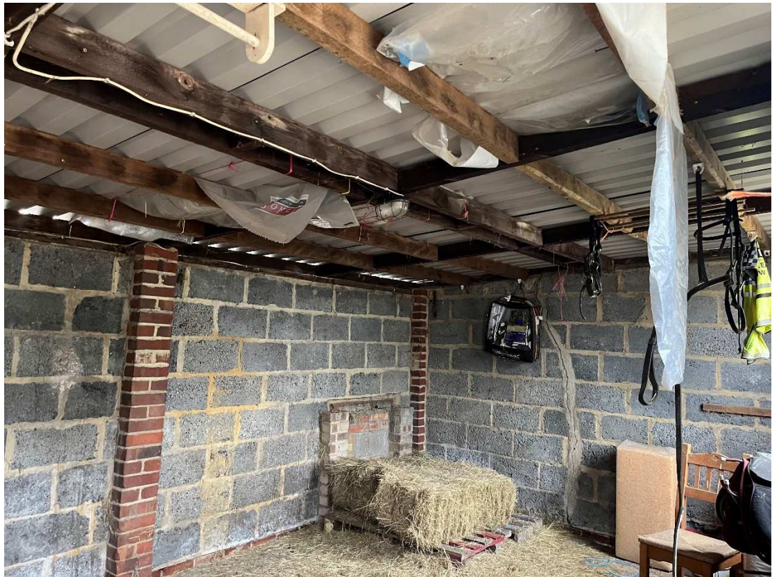
Figure 5. North Stable: Interior looking east.
