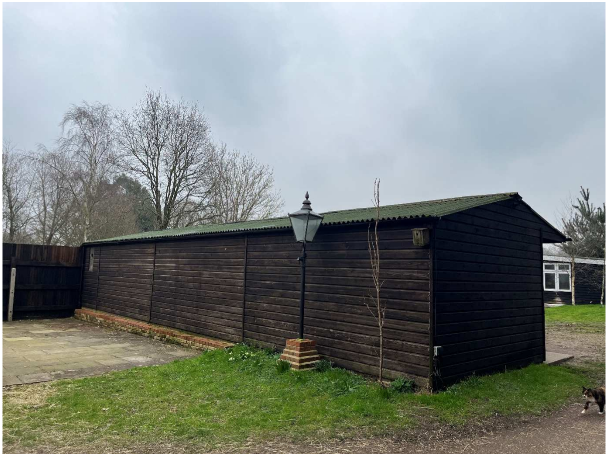
Figure 8. Building C eastern elevations.
