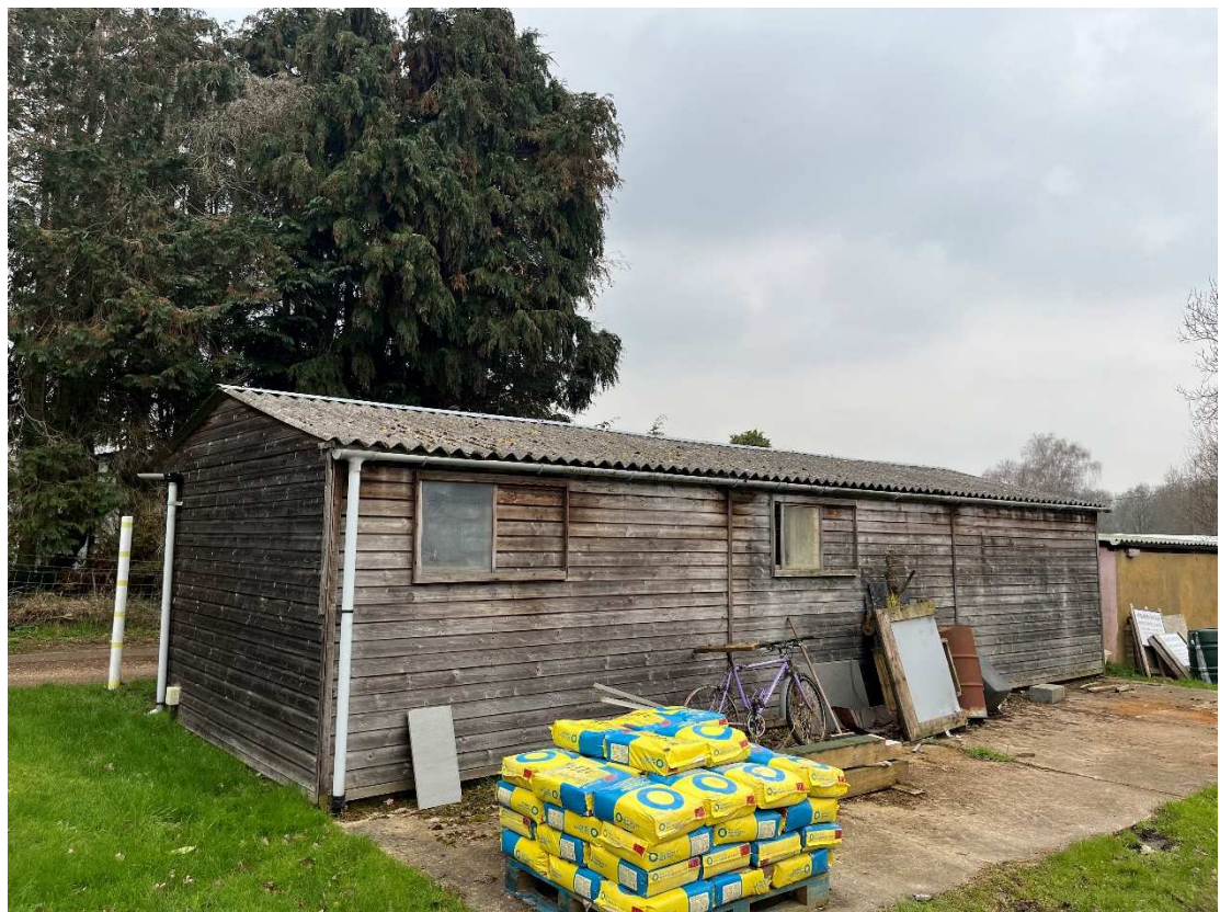
Figure 6. Building B: Eastern and southern elevations looking west.
