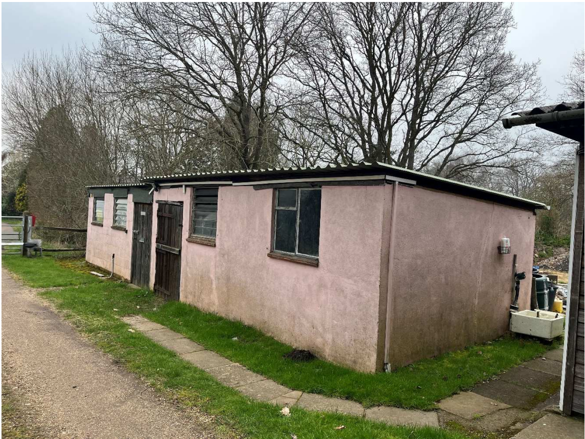
Figure 3. Building A: Western and southern elevations looking northeast.
