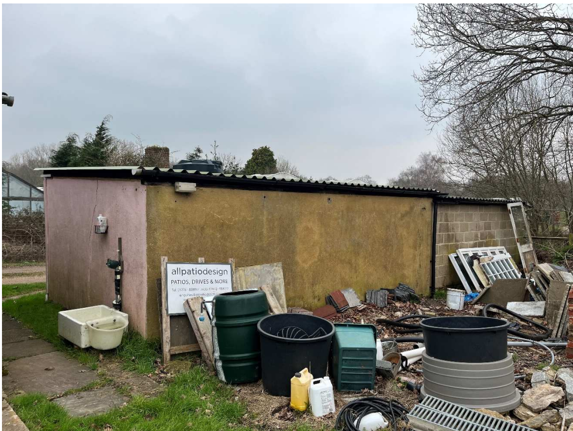
Figure 4. Building A: Eastern elevations looking northwest.
