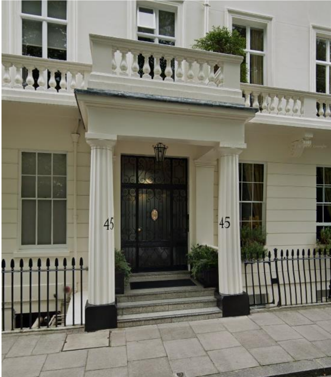
Photograph 1 – Existing Terrazzo / Tiled finish to front entrance steps.
