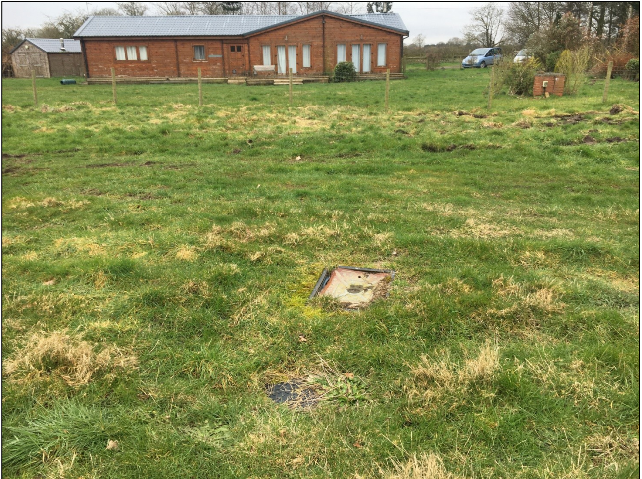
Figure 5 two drain covers in the survey area
