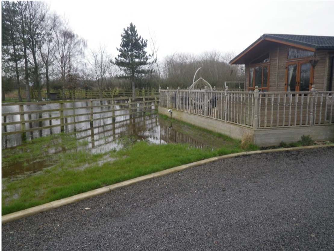
Plate 7 Looking northeast showing surface flooding in surrounding fields
