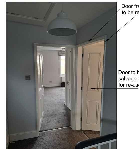
VIEW D: View of bedroom door from landing (door to be salvaged for re-use in new bedroom wall)
