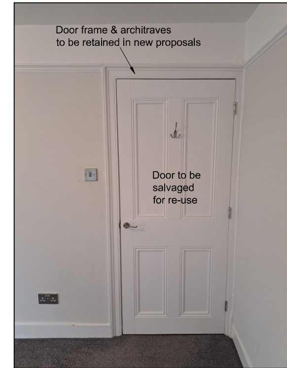
VIEW B: View of door from within bedroom (door to be salvaged for re-use in new bedroom wall)
